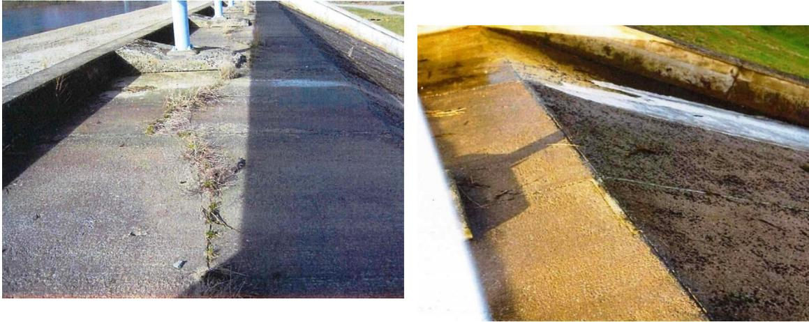
**Figure. B5 Historic crest cracking and isolated seepages on the left side on the chute**
