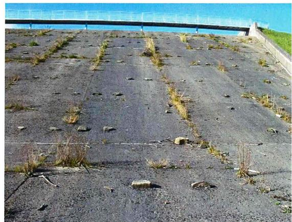
**Figure. B4 Well established vegetation on the crest slabs and on the chute in 2007**
