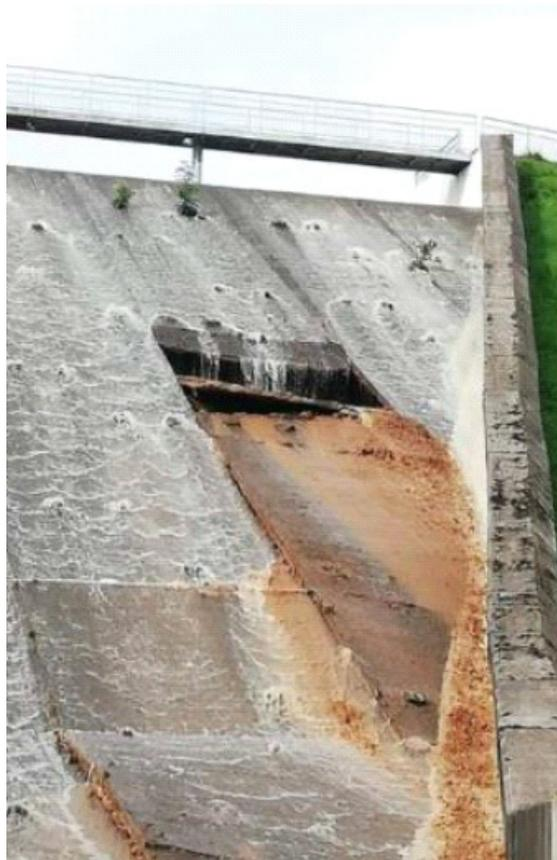
**Figure 5. Collapse of the First Slab into the Void (note the slabs that have been pushed up towards the foot of the spillway chute).**
