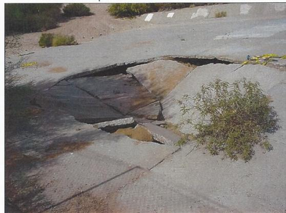
Figure 4.—Structural collapse of the slab system occurs when enough undermining has occurred to cause loss of support. This damage is typical of slabs placed on soil foundations (note: this slab is not reinforced so failure is more evident).
