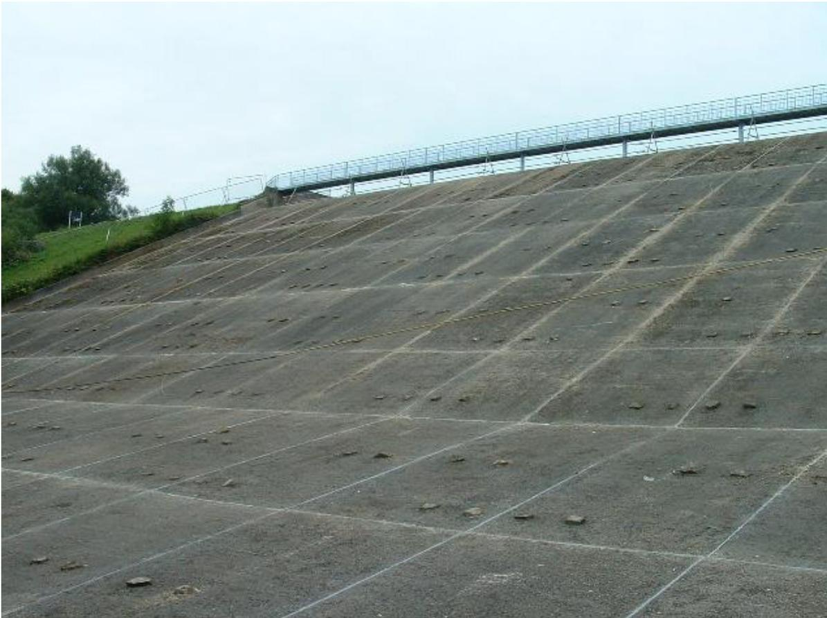
**Figure 9. Evidence of Good Maintenance with Joints cleaned out and Re-sealed, September 2008**
