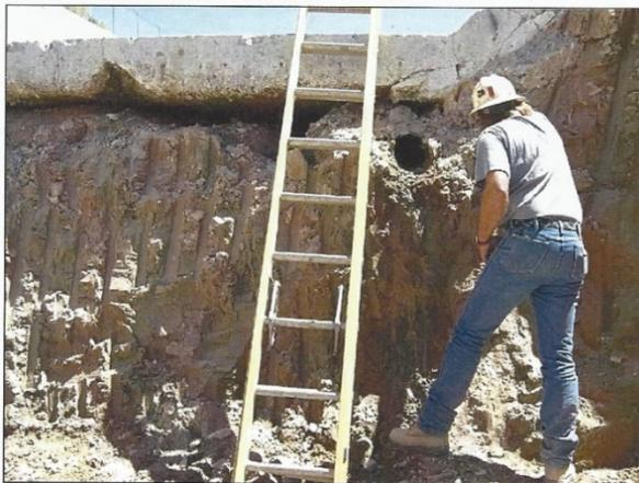
Figure 3.—Undermining of the chute slab has occurred due to flow entering at joints and cracks and transporting foundation material through unfiltered drains.
