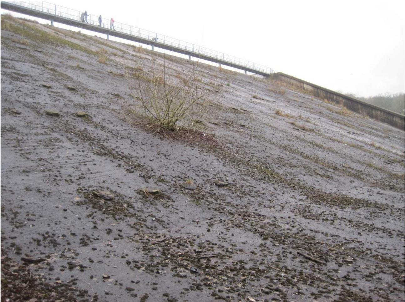
**Figure 10. Evidence of Poor Maintenance with Vegetation and Saplings Growing in Joints, January 2018**
