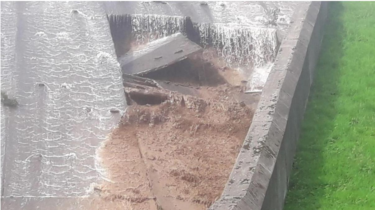
**Figure 6. Four Sections of Panels Collapsed into the Void**
