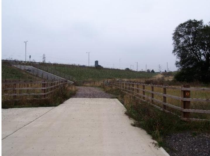
5.162 Other measures at J12 have been implemented, including signalisation of a number of crossings. **Figure 5.25** below shows the new overbridge footpath/cycleway crossing the M1, which has reduced severance across Harlington Road, where there was a previously blocked NMU access. Overall at J12 there has been an improvement for NMUs through provision of safer, signalised crossings and dedicated footways.
