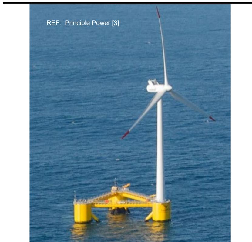
The design comprises a triangular base of floating cans with the turbine located directly onto one of the corners. The design has been proven to work at 2MW scale in the Windfloat Atlantic and Kincardine projects in Spain and Scotland respectively. A project is currently underway to implement a larger 8.4 MW turbine as an extension to the WindFloat Atlantic project.
