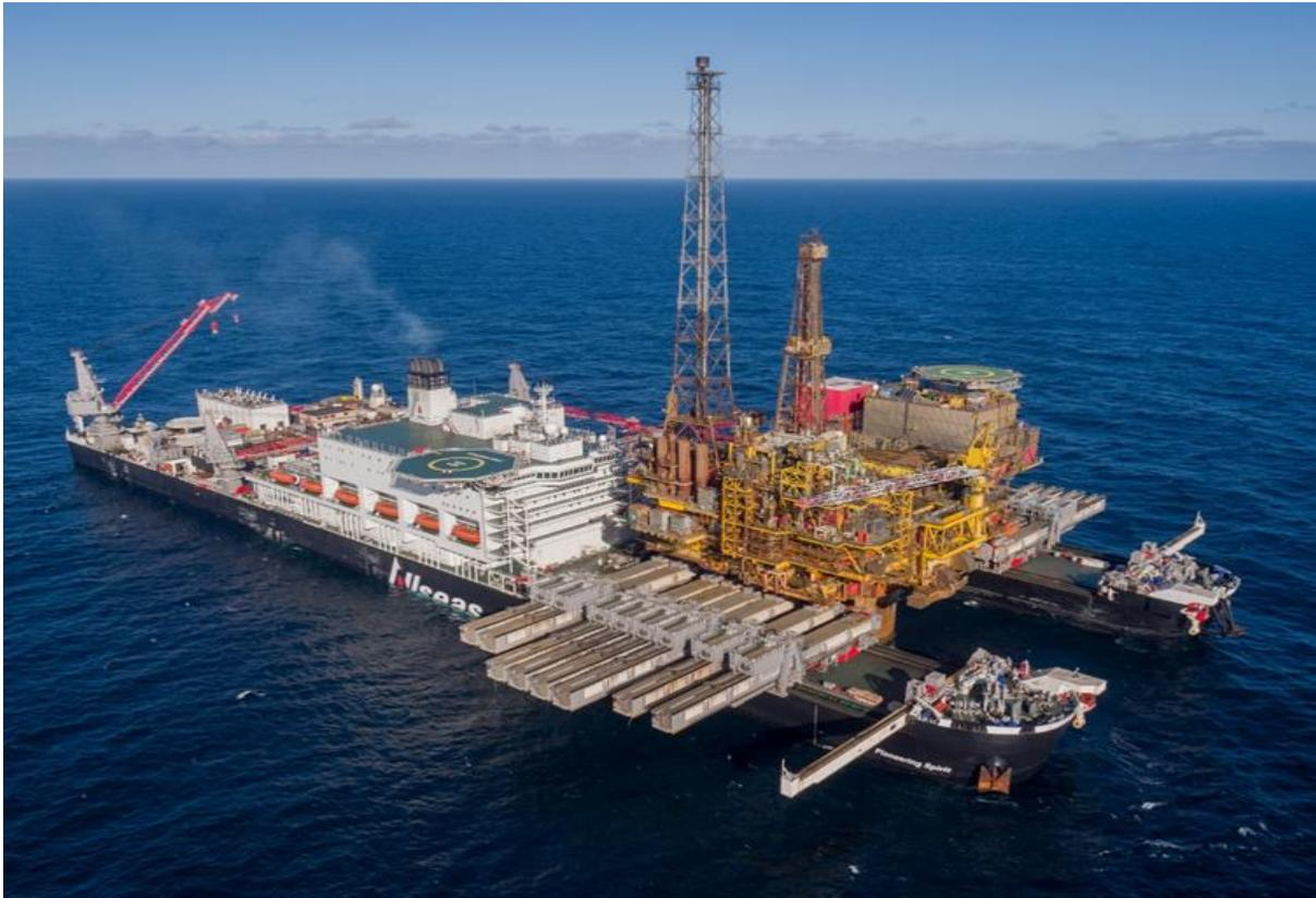
The SLV was stationed beneath the topside and the 16 large beams of the TLS (paired into 8 fork-lift units) were positioned under the prepared lift points on the underside of the PGDS (Figure 17). Each fork-lift unit had a yoke (lifting pad) that fitted on to one of the topside lifting points and was kept positively in touch with the topside by a hydraulic system that compensated for the movement of the vessel.
