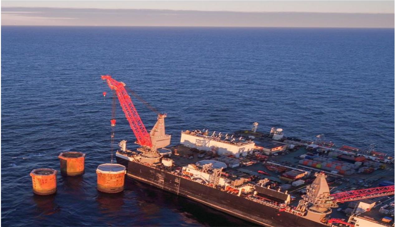
Figure 21. Condition of the Brent Delta GBS after removal of the topside and the fitting of leg caps and AtoN.
