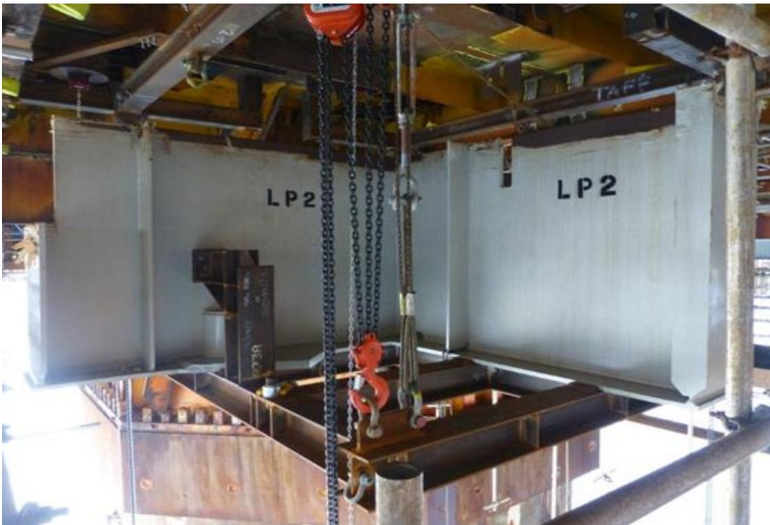
The topside required strengthening with additional steel in order to bear the forces that would be exerted during removal. A significant number of steel doubler plates were welded in place on the primary steel bulkheads of the Module Support Frame (MSF); this required the removal of some local obstructions.
