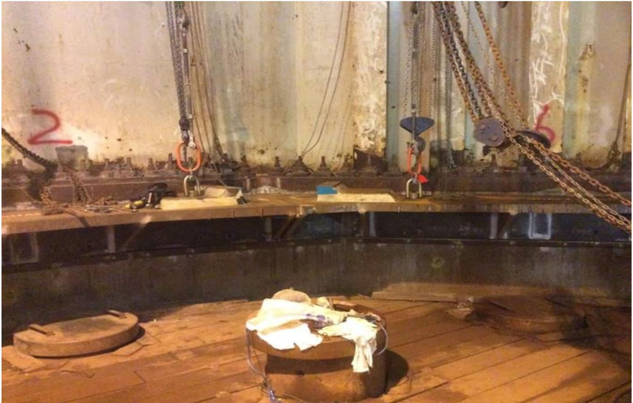
Allseas also identified four modules on the Module Deck where additional strengthening to the main steelwork was required. Again, some removal of local obstructions was required before the stiffeners could be welded in place.
