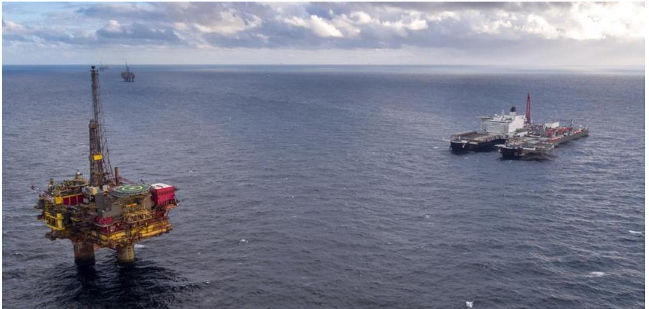
The vessel was accurately positioned so that the GBS legs fitted into the vessel’s slot (Figure 16); the clearance between the vessel’s hull and the platform substructure was sufficient to allow for some movement of the vessel. The beams of the Topside Lifting System (TLS) were fully retracted to provide the maximum clearance between the SLV and the substructure when manoeuvring. Positioning was achieved by using a combination of the *Pioneering*
