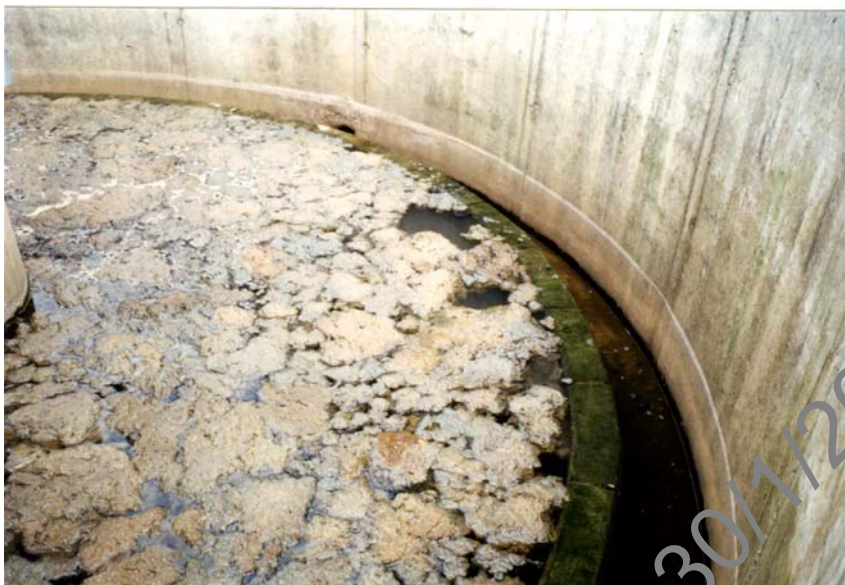
Plate 2.12: Rising sludge as a consequence of denitrification within the settlement phase of an activated sludge system treating leachate, Germany, 1990
