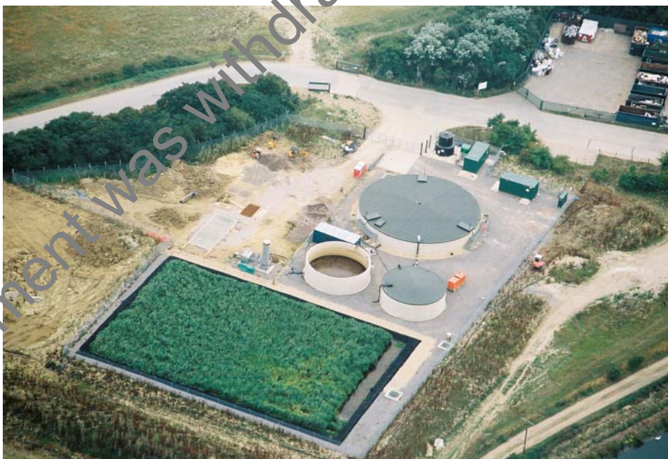
Plate 2.21: Efford Leachate Treatment Plant, Hampshire, showing horizontal flow reed bed used to polish SBR effluent.
