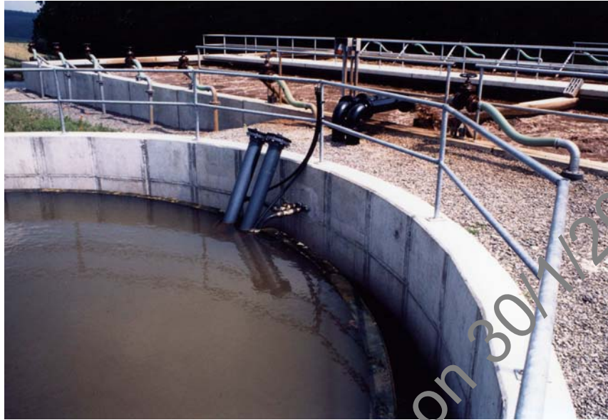
Plate 2.11: Typical application of the activated sludge process to leachate treatment, showing sludge settlement in the foreground, and aerobic reactor in the background, Germany, 1990
