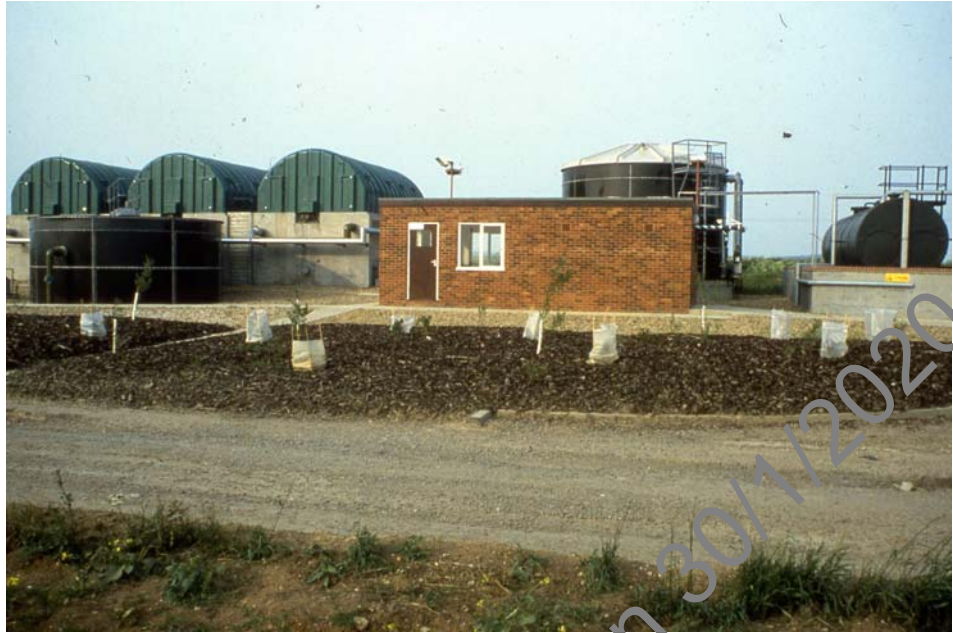
Plate 2.18: Pitsea RBC Plant
