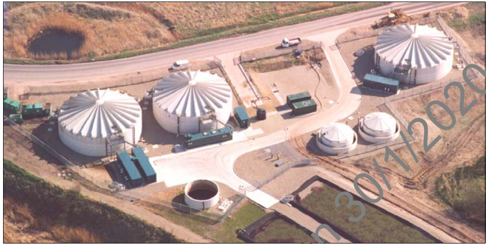
Plate 2.16: Large tank-based SBR System: Arley Landfill, Warrington, 450 m 3 /d (COD 10,000 mg/l, ammoniacal-N 2500 mg/l), 2001- (see Robinson and Last, 2003)
