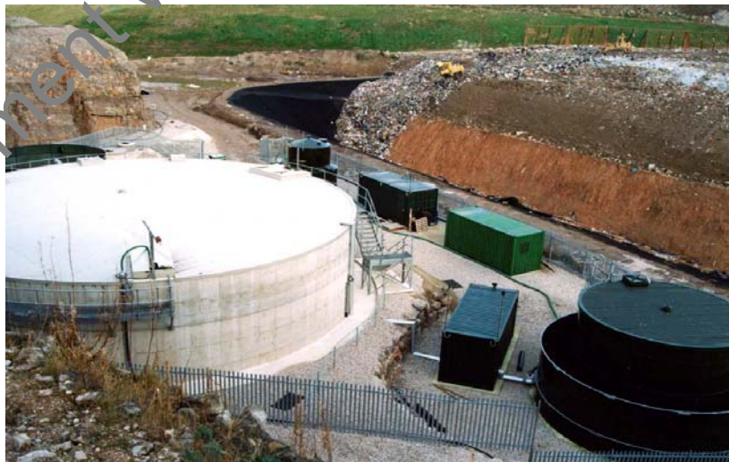
Plate 2.15: Typical example of an above-ground SBR leachate treatment system: Llanddulas Landfill, Abergele, 150 m 3 /d, 2002- (see Robinson and Last, 2003)
