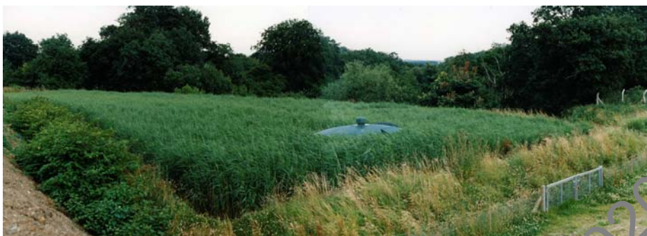
Plate 2.20: View of the Monument Hill Landfill horizontal flow reed bed system for direct treatment of weak leachate, 1993.
