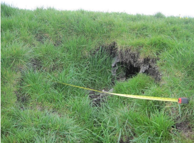
Photo 6: Sink hole near the dam crest
