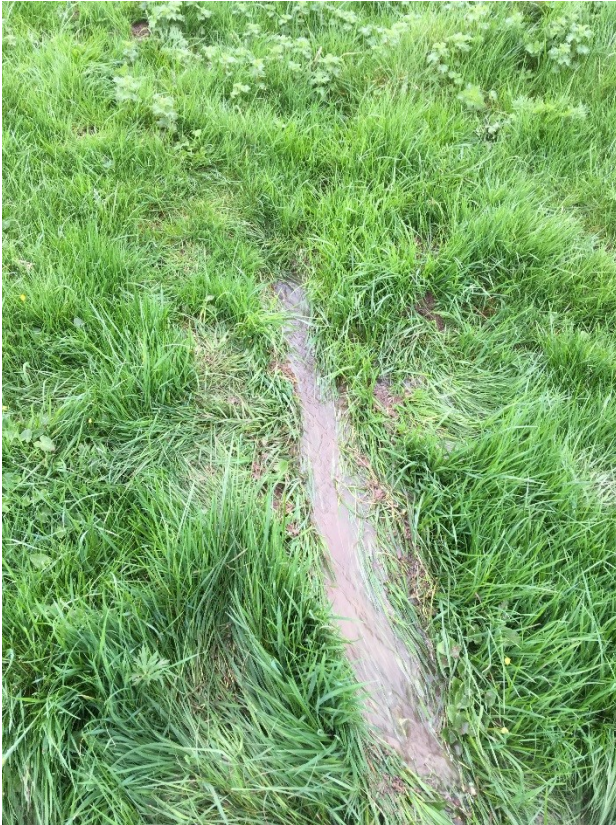
Photo 5: Leakage from animal burrow
