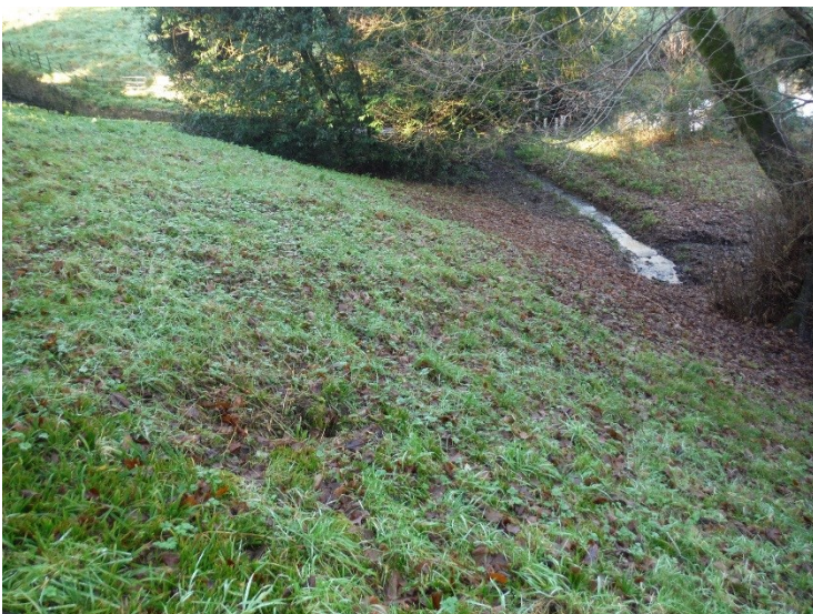
Photo 8: Leakage from the embankment right mitre
