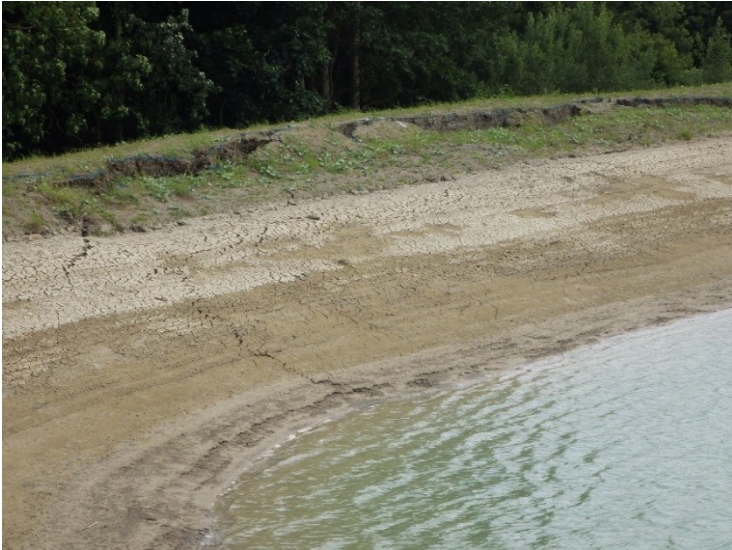
Photo 3: Slip failure in the inner shoulder of the embankment due to rapid emptying of the reservoir
