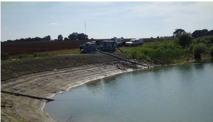
Photo 2: Reservoir being emptied by pumping
