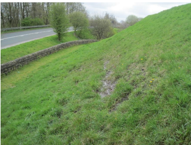
Photo 7: Line of seepage on the downstream face
