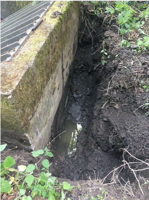
Photo 4: Excavation of fill adjacent to conduit headwall
