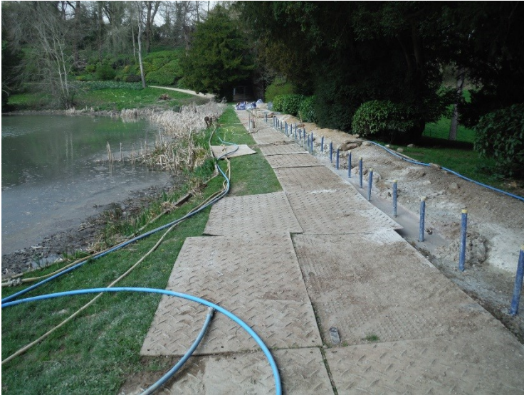
Photo 9: Grouting works to remediate and improve the embankment using the tube-à-manchette method.
