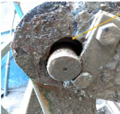
Figure 11: erosion of hinge pins and holes on New Bow sluice
