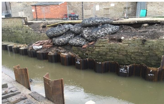
Palmer's Brewery wall failure
