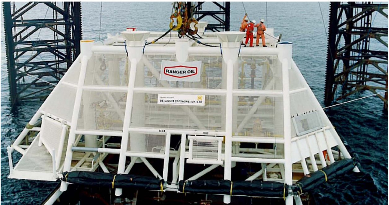
Figure 2.2 Anglia West (B) Subsea Manifold
