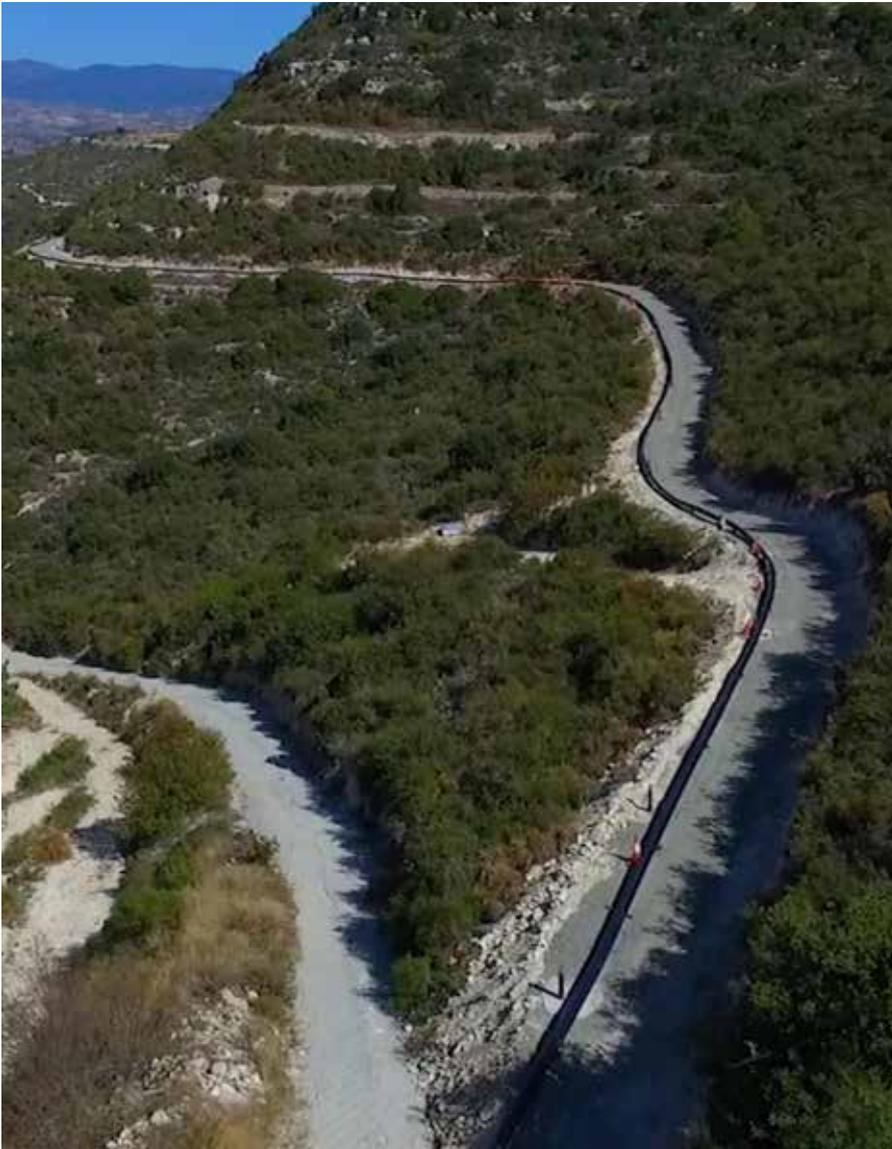
The 532m HDPE pipeline prior to insertion in the tunnel © Infrastructure Service Provider Cyprus
