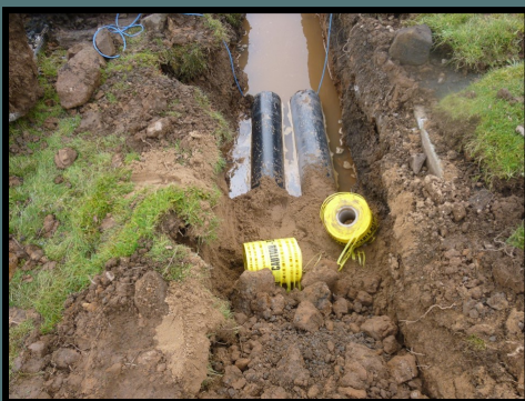
Our excavations RIE has dramatically reduced the time it takes to start digging
