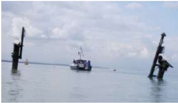
Photograph of the wreck during 2013 hull thickness survey.
