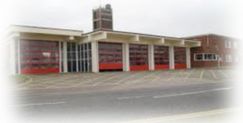
Bedford Fire Station
