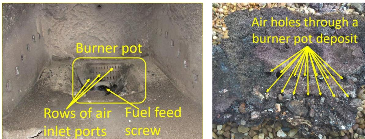
Figure 32: The burner pot and an example of ash deposits removed from burner pot
