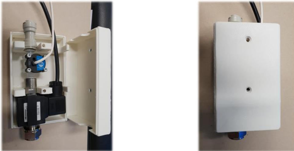
Figure 8 - Valve and meter secure housing
