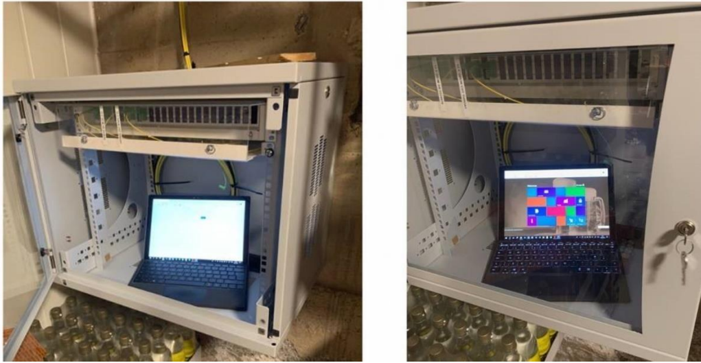
Figure 22 – Example of a typical back-office server enclosure
