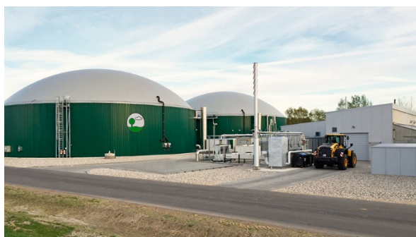
Figure 16 Farm-scale AD plant
