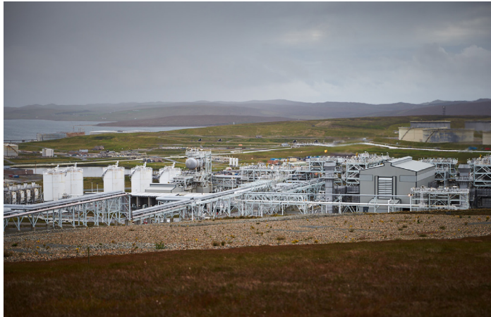
Shetland Gas Plant
