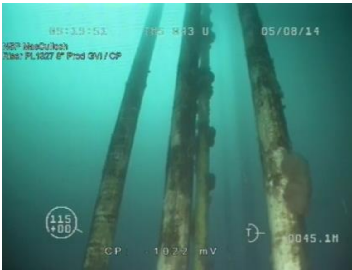
Figure 4.8: Representative example of ROV video footage showing presence of L. pertusa on PL1327
