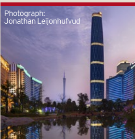
Photograph: Jonathan Leijonhufvud The Guangzhou International Finance Centre – designed in the UK by Wilkinson Eyre Architects – uses 20 percent less steel than similar skyscrapers.
