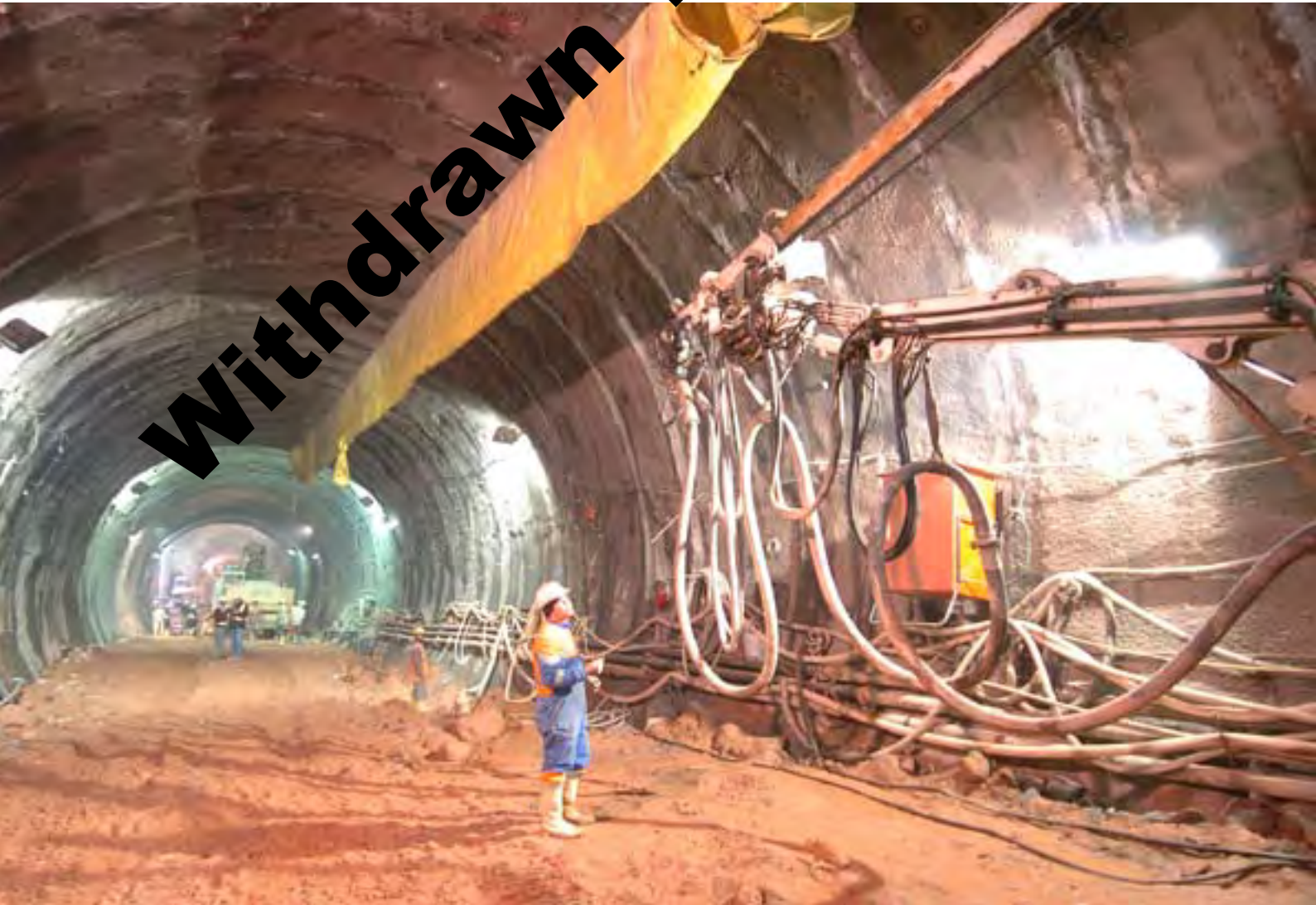
Tunnel under construction
