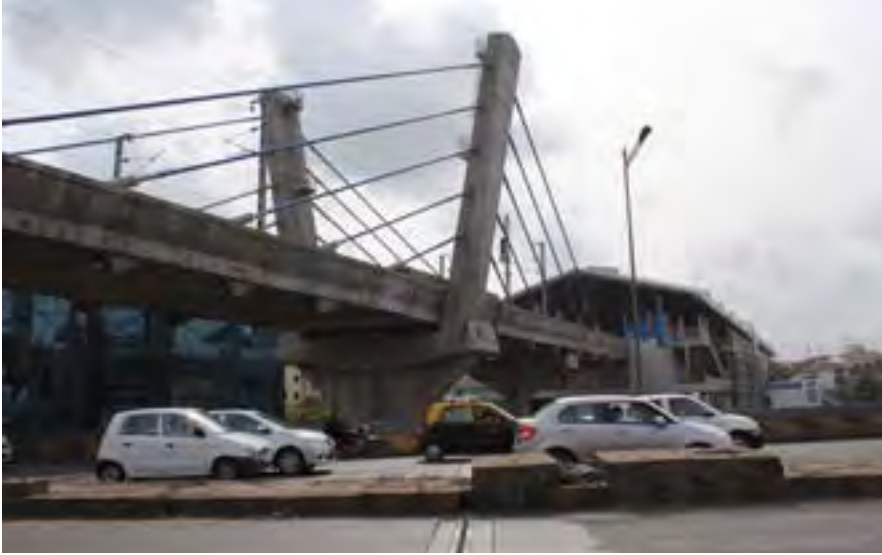
Mumbai Metro station under construction
