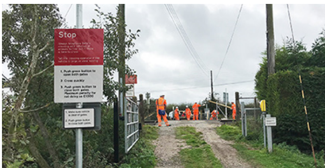
The UWC with power operated gates at Frogal Farm, Kent
