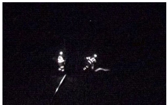
Narrowly avoided collision between an express passenger train and two staff who were preparing to apply earthing straps to the overhead line
