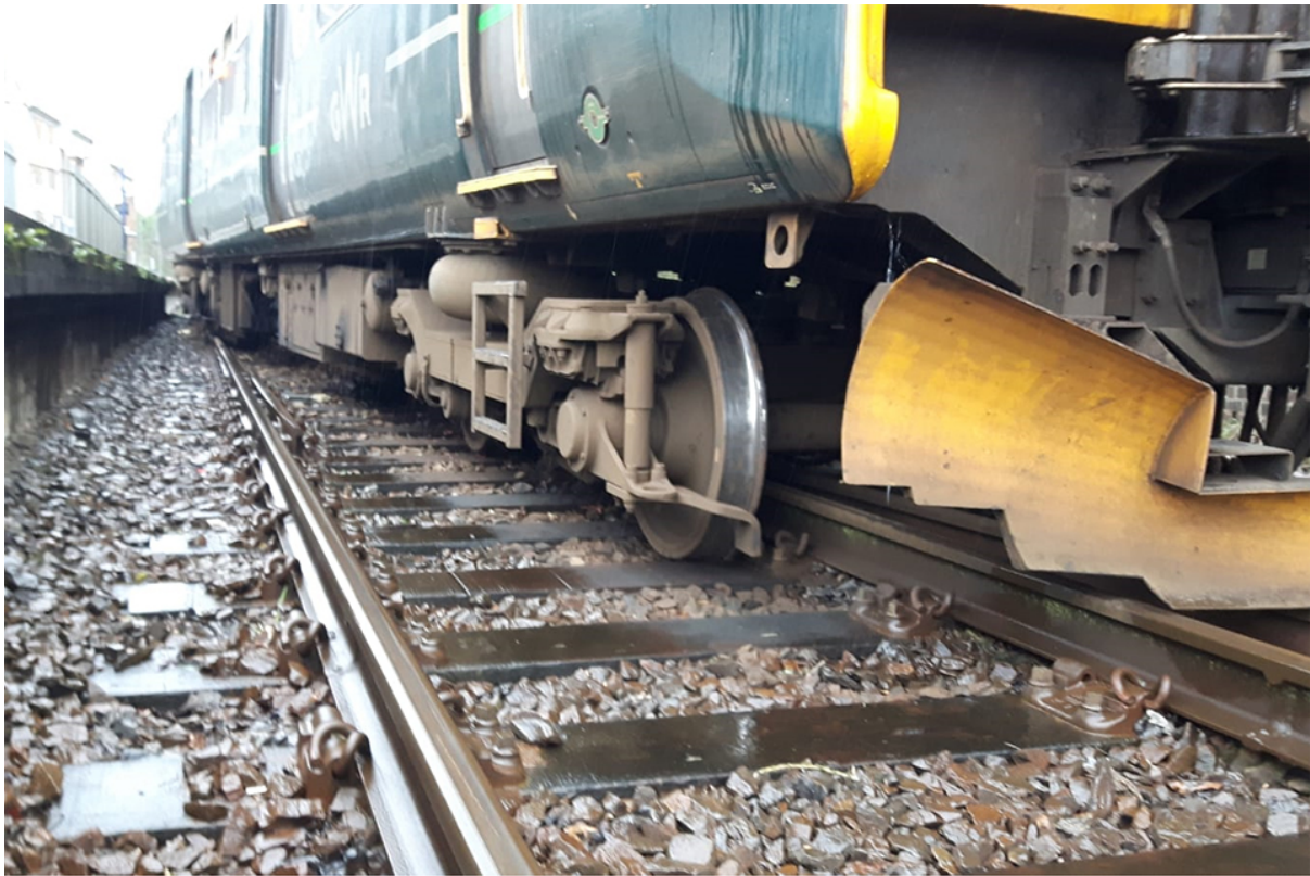
Figure 2: The derailed train 2T76
