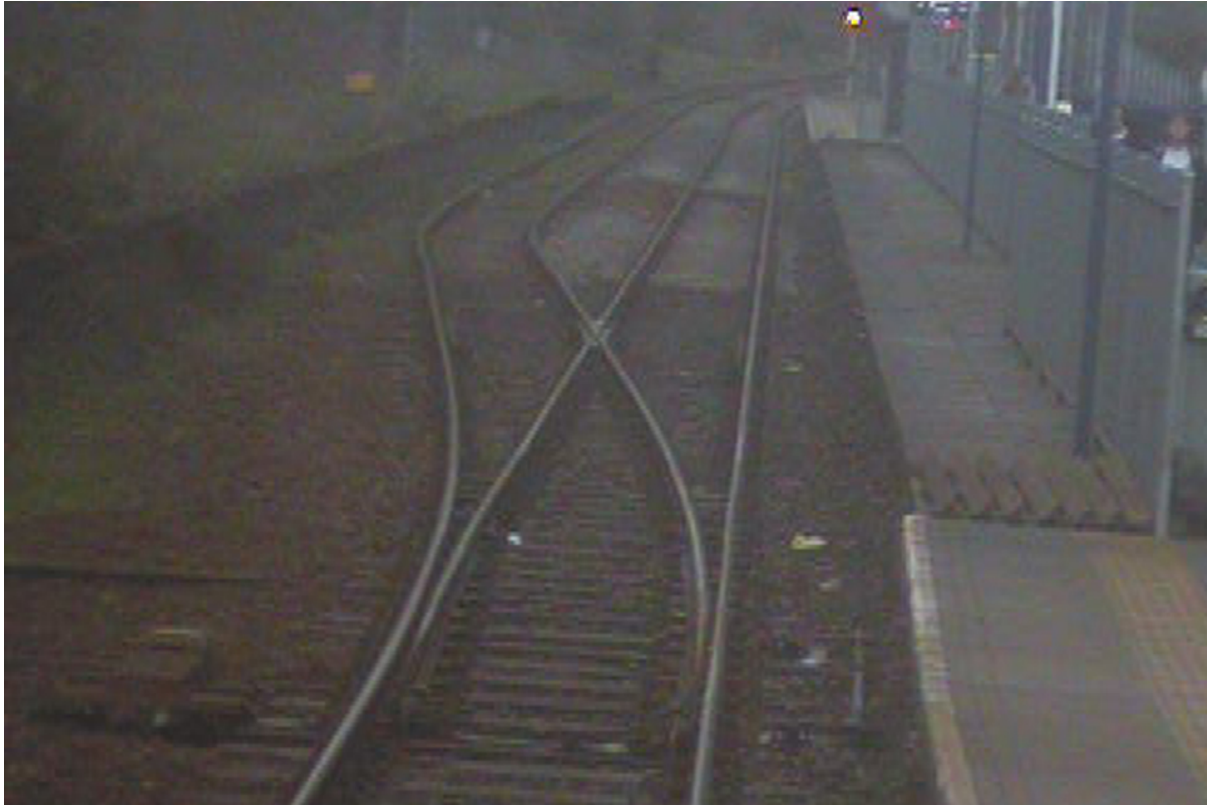
Figure 4: Forward Facing CCTV image from train 2T76 showing points 27 lying in the mid-position at Penryn station
