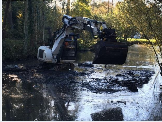
An excavator on individually operated legs was able to remove sediment from within the pond.
