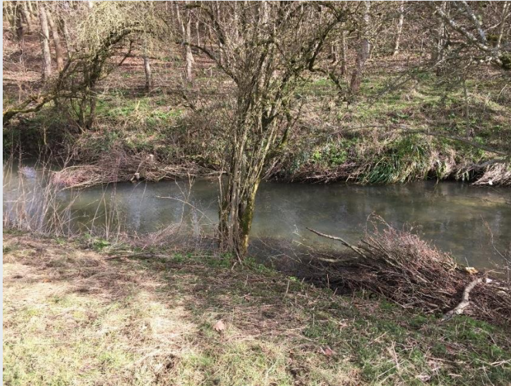
Alternate berms constructed to re-form a meander within the banks of this straightened section
