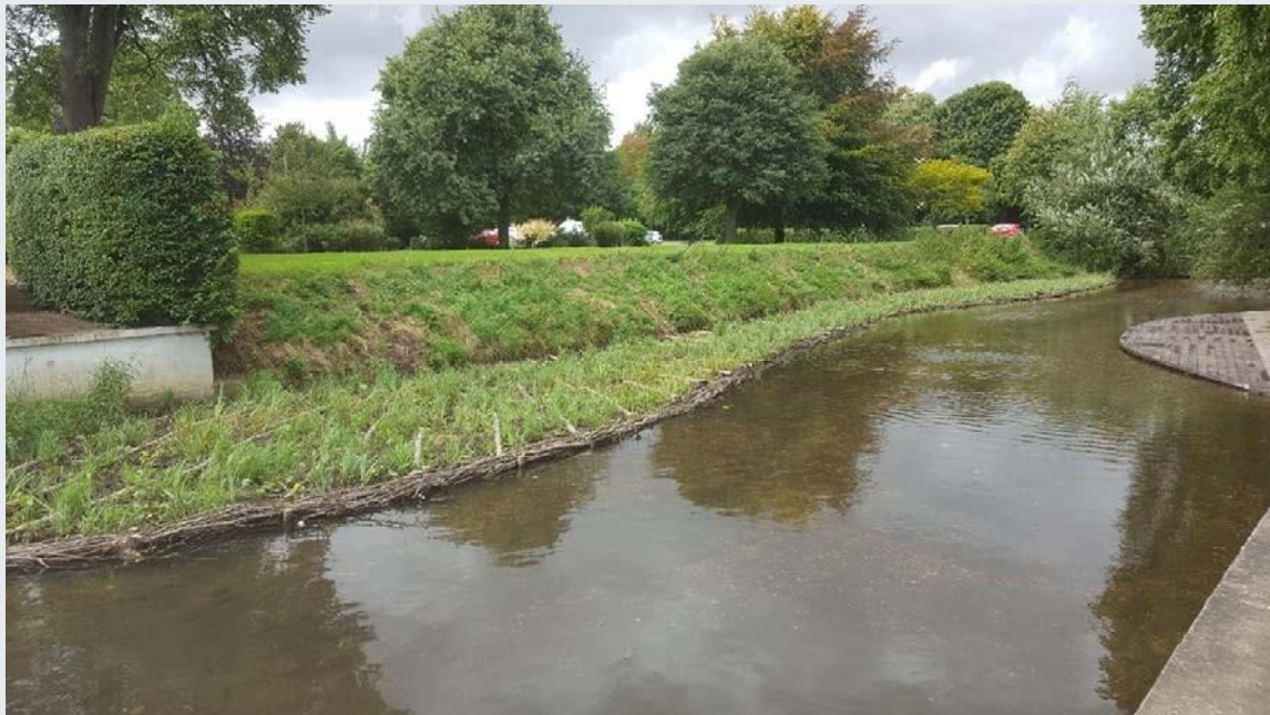
Wyndham Park berm creation and improvements
