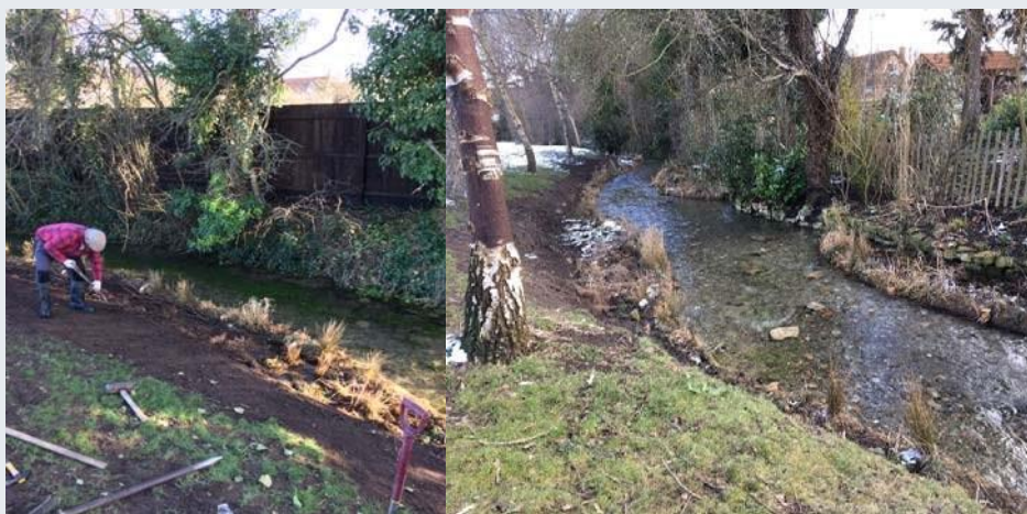
Welton Beck Project under construction and the completed design
