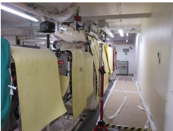
Neutron detector in various locations outside contaminated gloveboxes, measuring the fissile content inside
