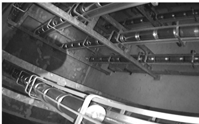
Endoscope images of the internal spaces in a store, the packages can be seen in open racks
