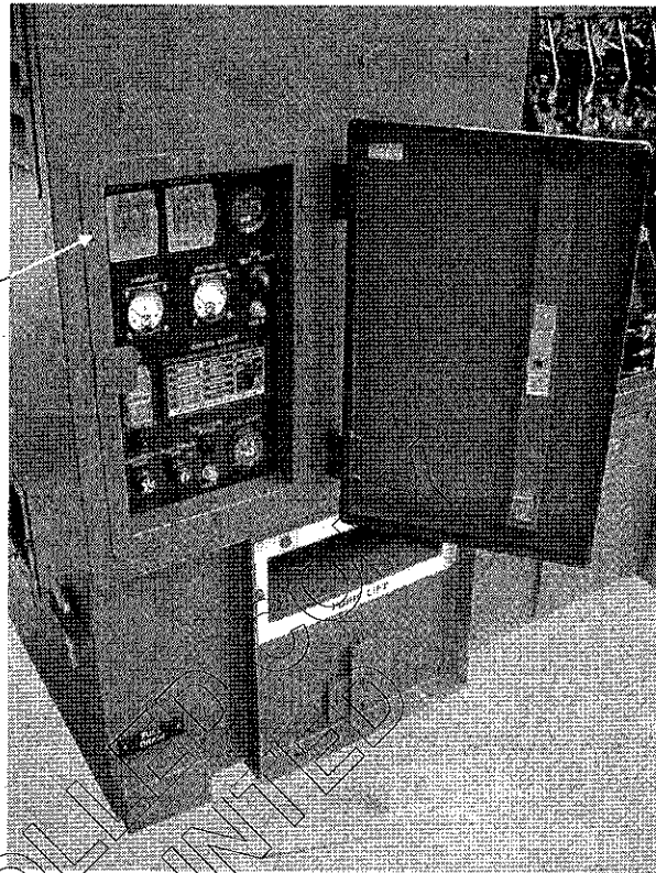
Fig 3 Control panel and door
