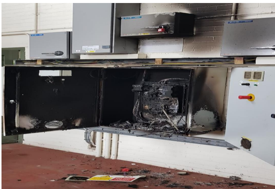
Photograph 1 showing the damage resulting from the overheating of the electrical Inverter Drive Motor
