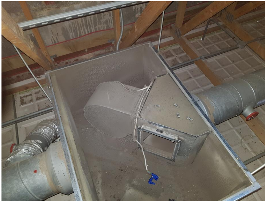
Photograph 2 showing dust build-up in the Air Handling Unit
