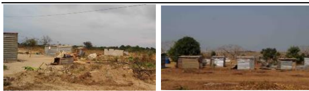
Figure 5.2 Temporary Residential Structures
