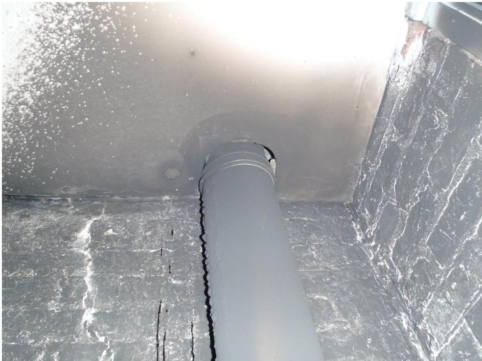
**Figure 34 - Inadequate fire stopping around soil pipe penetrating compartment floor**
