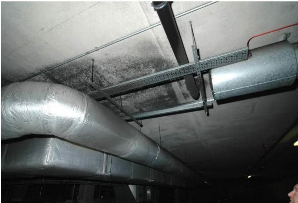
**Figure 35 - Flow from impulse jet fan obstructed by HVAC ducting**
