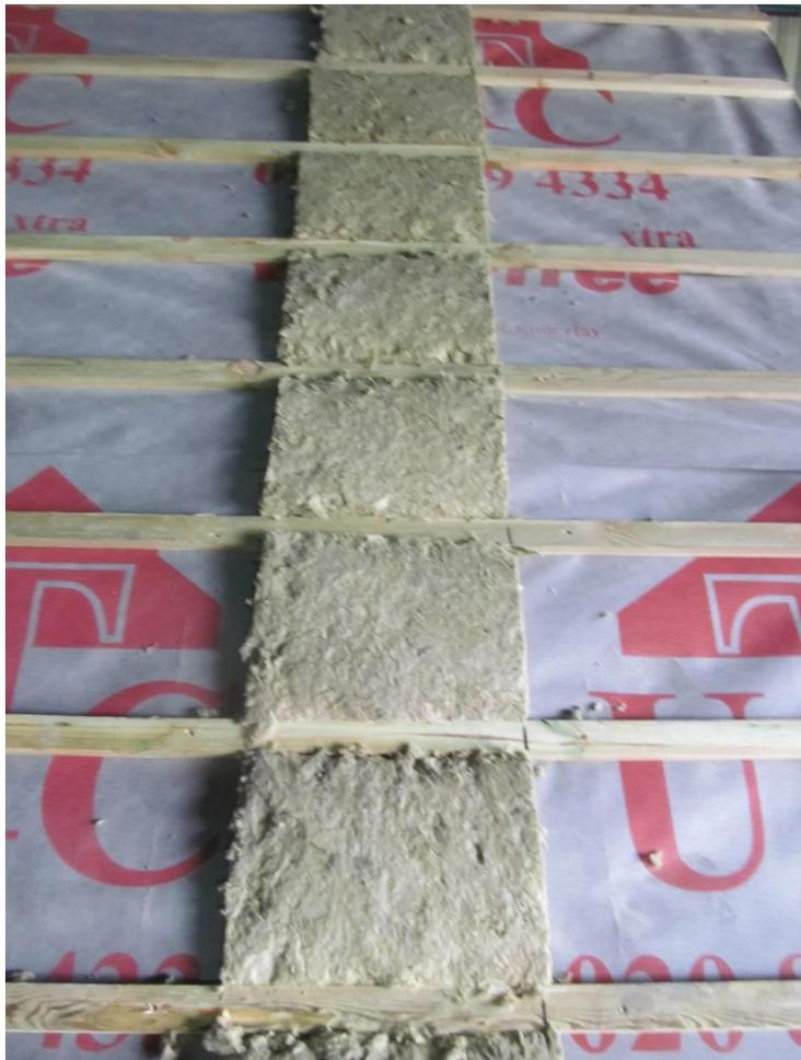
**Figure 17 - Insulation between tiling battens prior to fixing roof tiles**
