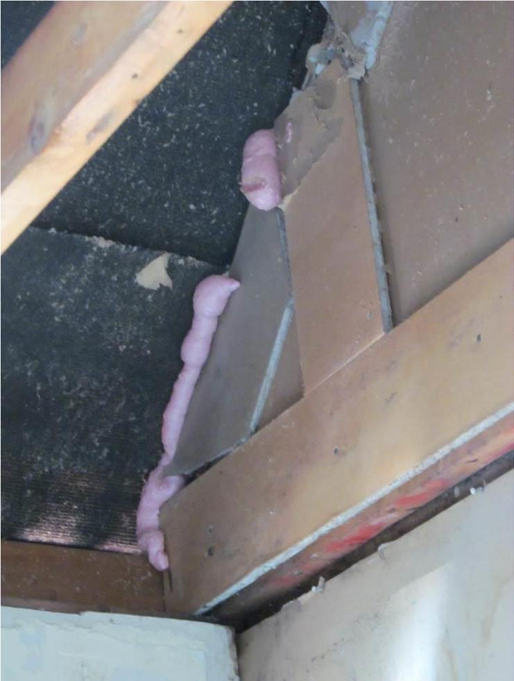
**Figure 12 - Sealing between compartment wall and roof construction**
