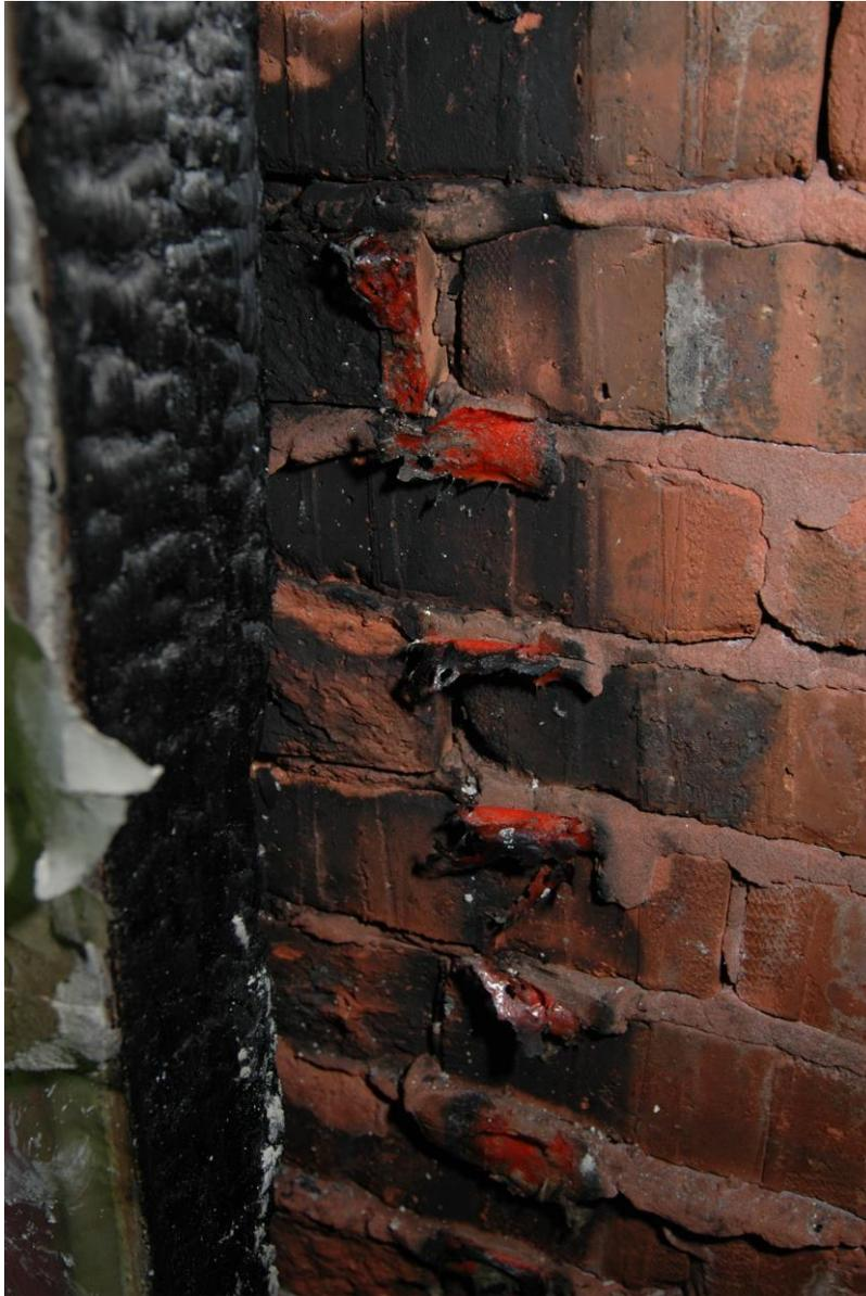
**Figure 29 Remains of cavity barrier on external wall**
