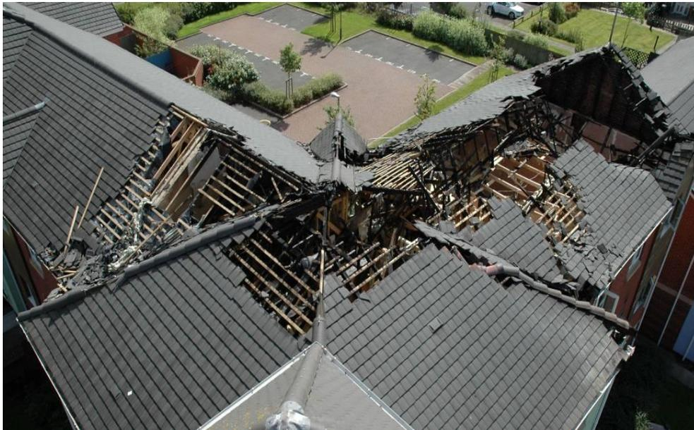
Figure 9 - Aerial view showing damage to roof structure
