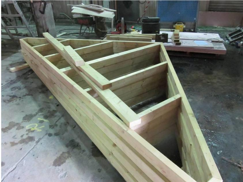
**Figure 14 - Timber used to form spandrel panels**
