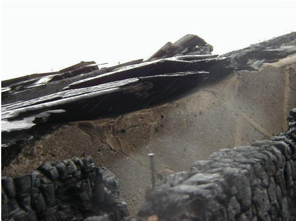
Figure 3 - Lack of fire stopping between compartment wall and roof covering
