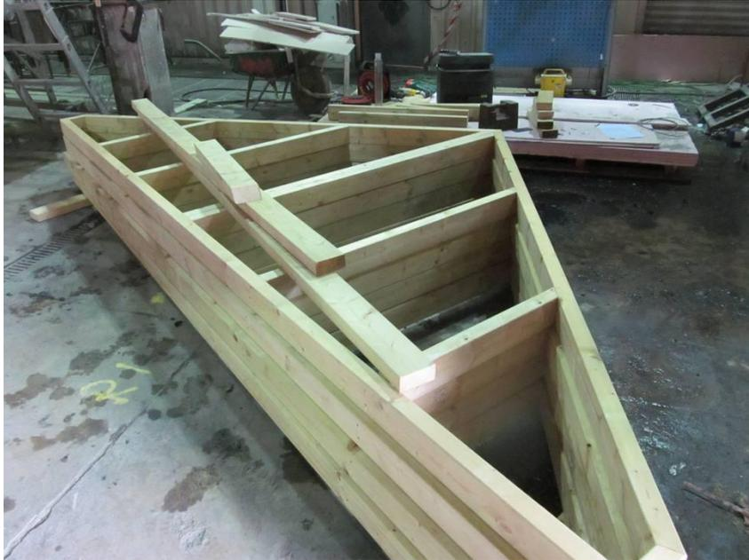
**Figure 2 - Timber used to form spandrel panels**
