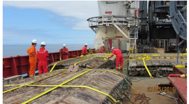
Figure 9.3.1: Mattresses Recovered and Secured on-deck
