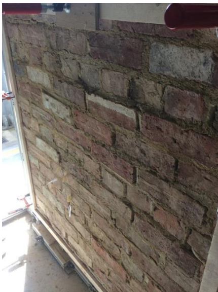
Figure 33: At the construction stage, each wall was built within a wooden frame which could be removed allowing the moving frame to be attached. The wooden frame can be seen surrounding this wall (Wall 4, built with an English Garden Wall Bond).
