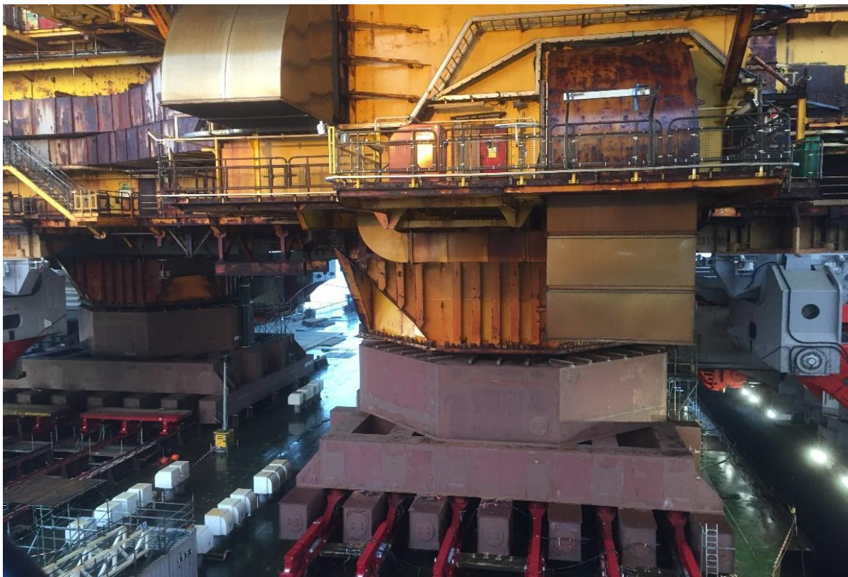
Figure 26. Transferring the Brent Delta topside from the Pioneering Spirit to the Iron Lady.
