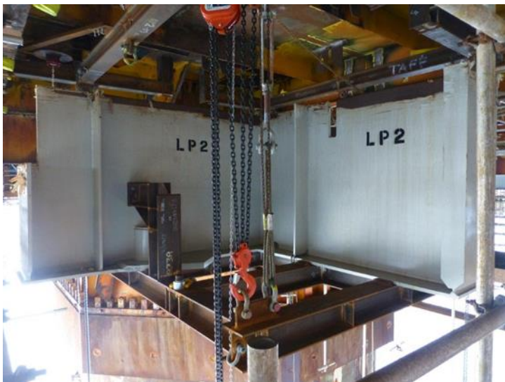
Figure 7. A Cruciform Strengthening Beam in Place under the PGDS on Brent Delta.
