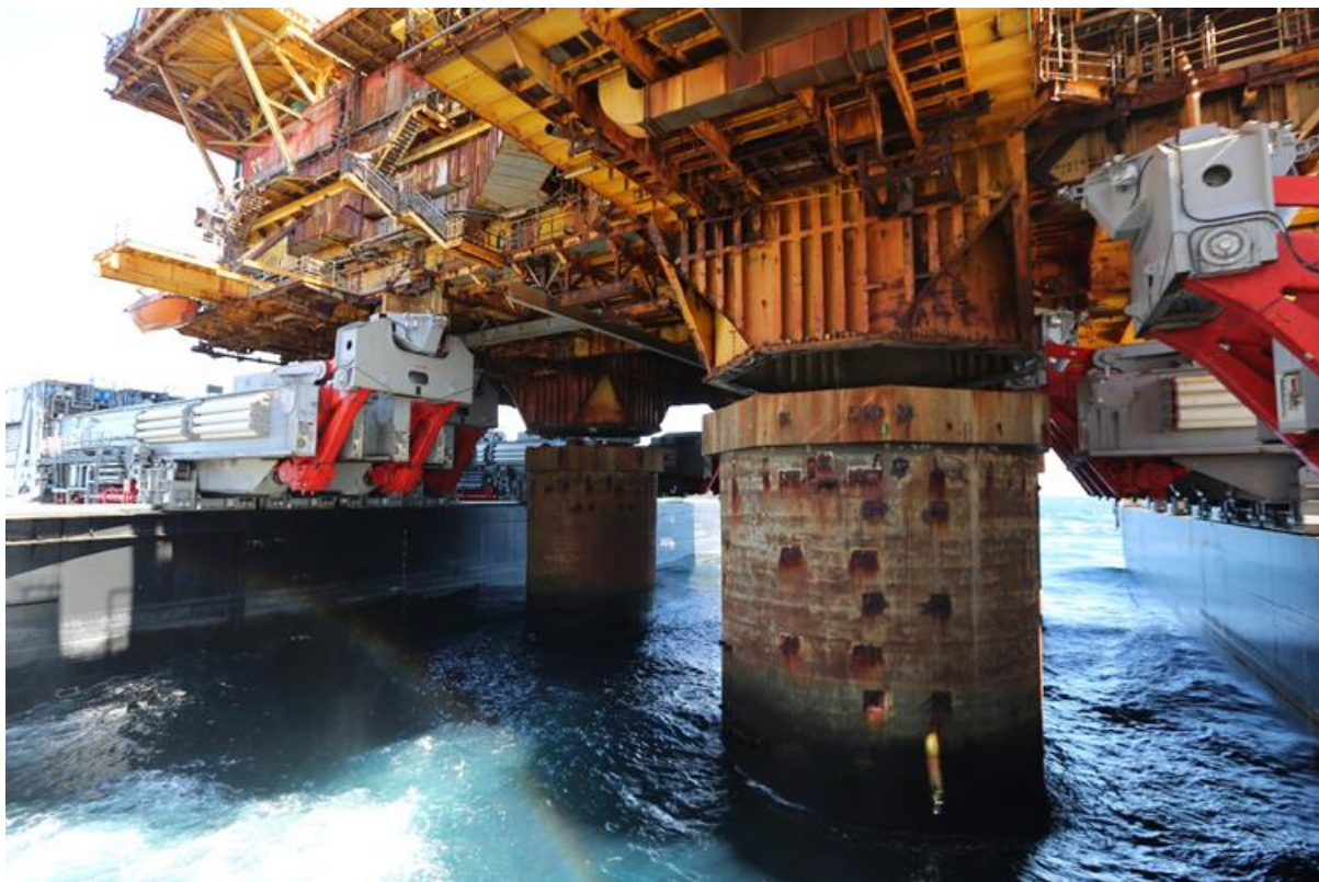
Figure 18. Brent Delta Topside Lifted Clear of GBS legs, April 2017.
