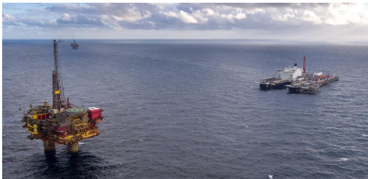
Figure 15. The SLV Pioneering Spirit aligning with the Brent Delta platform.
