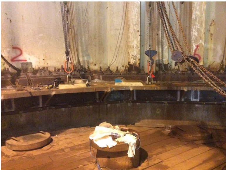
Figure 9. Shear Restraint Fitted Inside a Leg on Brent Delta.
