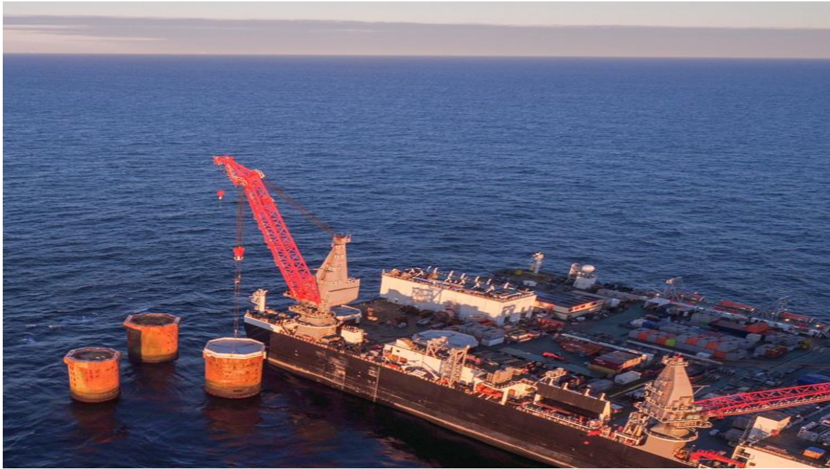
Figure 20. Fitting the Concrete Caps and AtoN to the Brent Delta GBS Legs, April 2017.
