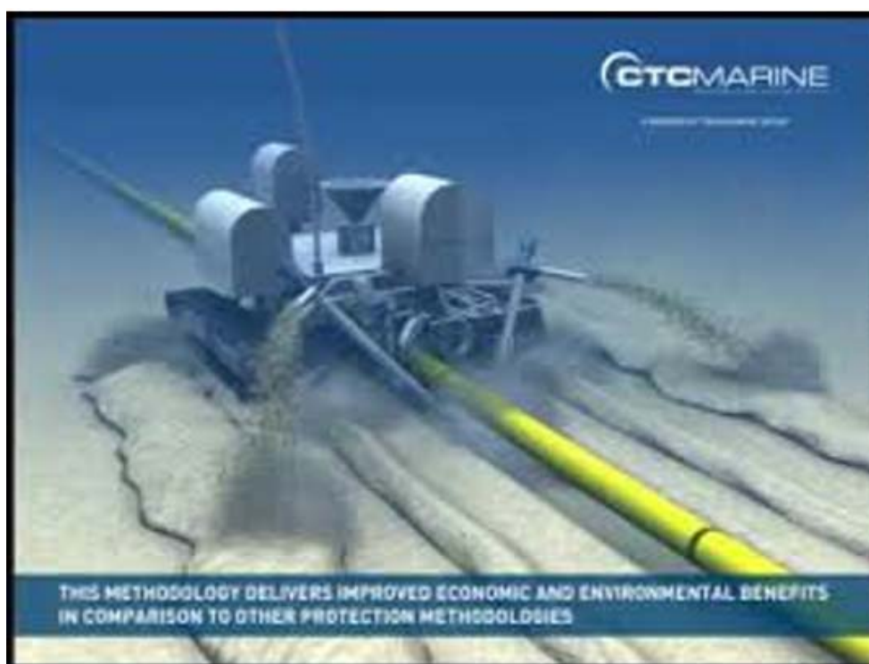
Figure 2.1 Burial of Pipeline using Jet Trenching
