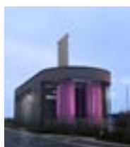
Front cover image credit: Gateshead Energy Centre WSP Parsons Brinckerhoff
