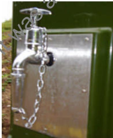
All service reservoir compartments should be fitted with individual sampling taps in order that the microbiological quality of water within each compartment can be determined.
