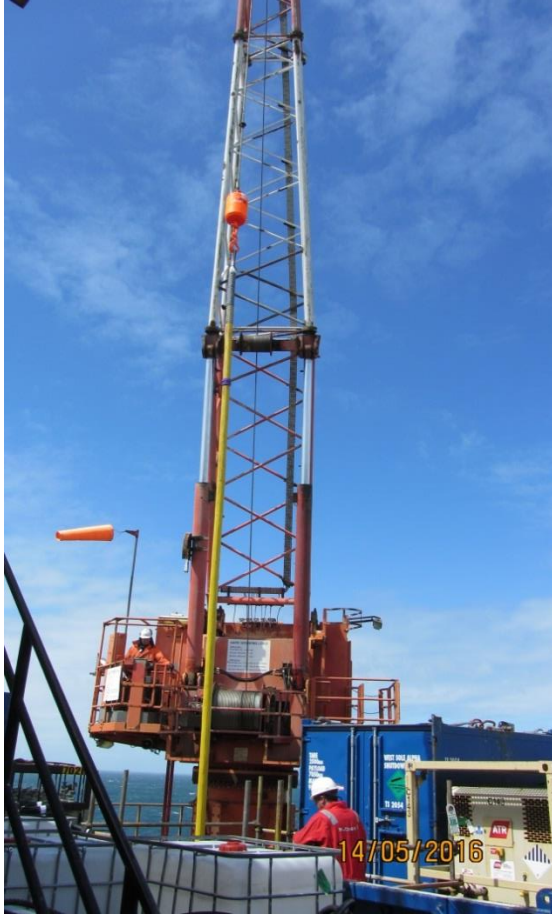
Figure 9.4.1: Umbilical lifted through J-tube using A2D platform crane
