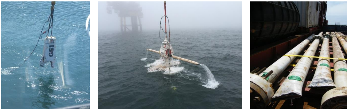
Figure 9.3.1: Pipeline section cut, recovered using grab, and stored on deck
