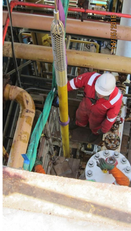
Figure 9.4.1: Umbilical lifted through J-tube using A2D platform crane
