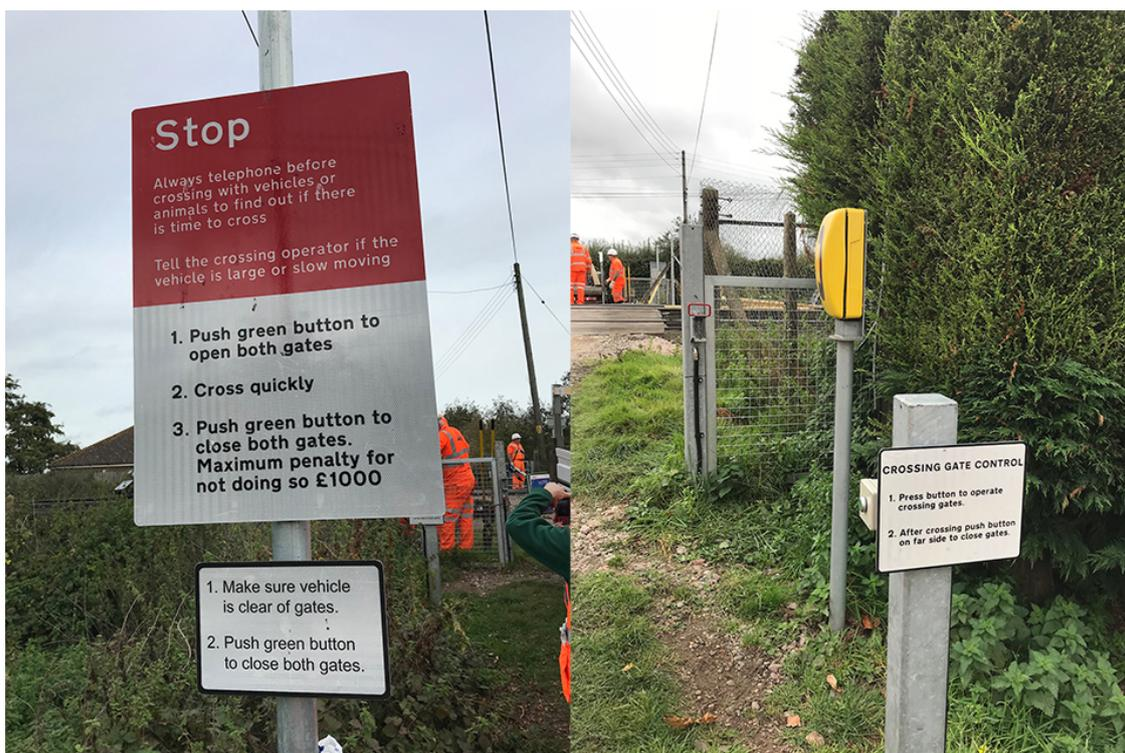
The signs at Froggnal Farm crossing, showing the instructions to vehicle users (left) and the telephone cabinet, gate operating button and subsidiary instruction sign (right)<sup>13</sup>
