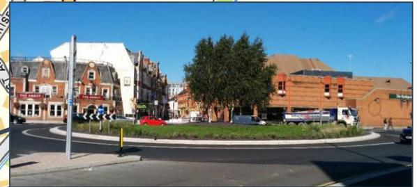
Footway widened outside the station. Guard rail removed. Roundabout made smaller to improve line of sight between station and town centre.
