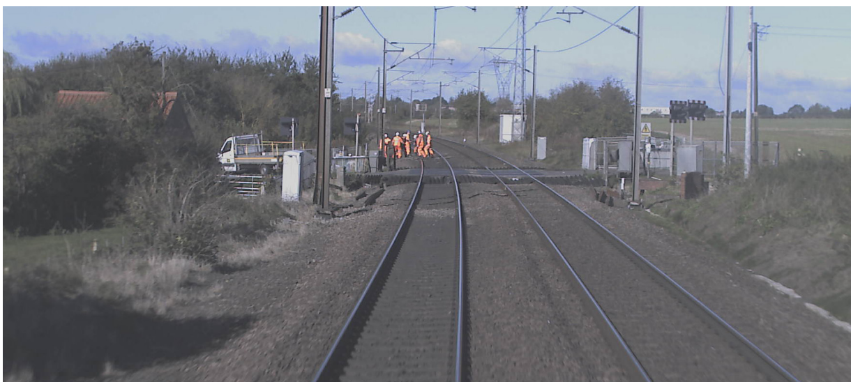
Figure 6: Forward facing CCTV image from train 1D09 showing three workers on the track as it approached the group on the Down Main line approximately 2 seconds before reaching the site of work (image courtesy of Virgin Trains East Coast)
