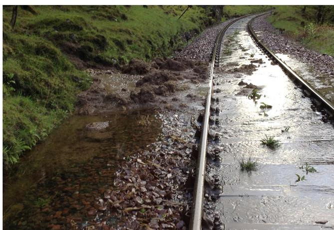
*Figure 13: view of minor landslip which occurred in June 2015 about 150 metres west of the 2018 accident landslip (photograph courtesy of Network Rail)*
