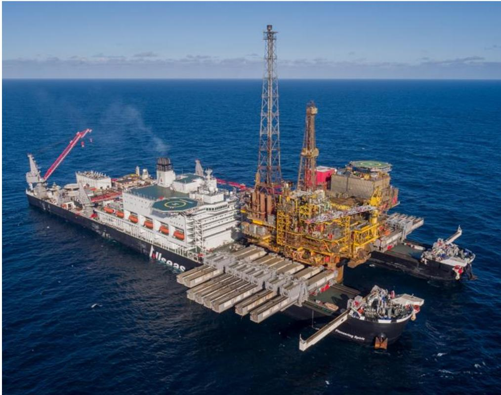
Figure 11 Fitting the Concrete Caps and AtoN to the Brent Delta GBS Legs, April 2017
