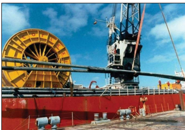
Cut pipeline sections
