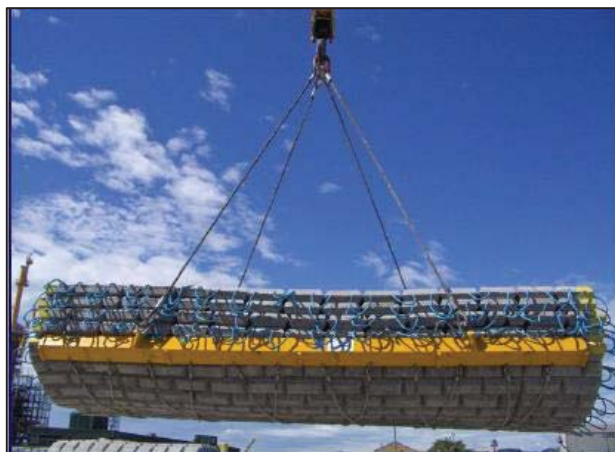
Concrete mattress lifting frames (speed loaders)
