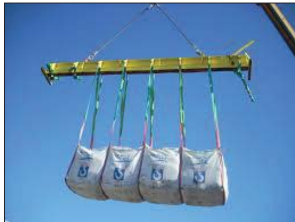
Rock-filled FIBC deployment
