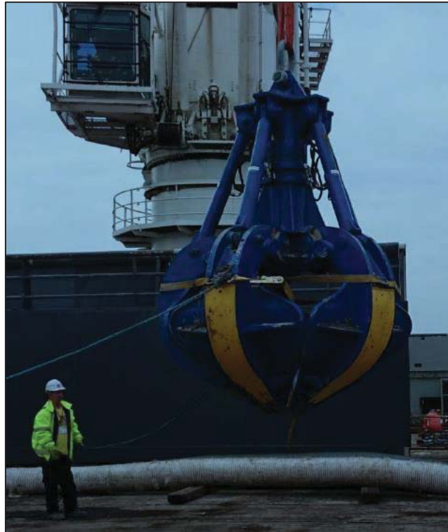
Mattress lift using grab
