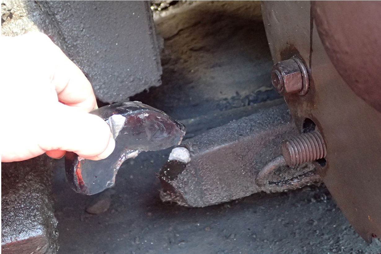
The equalising beam with the detached hook end
