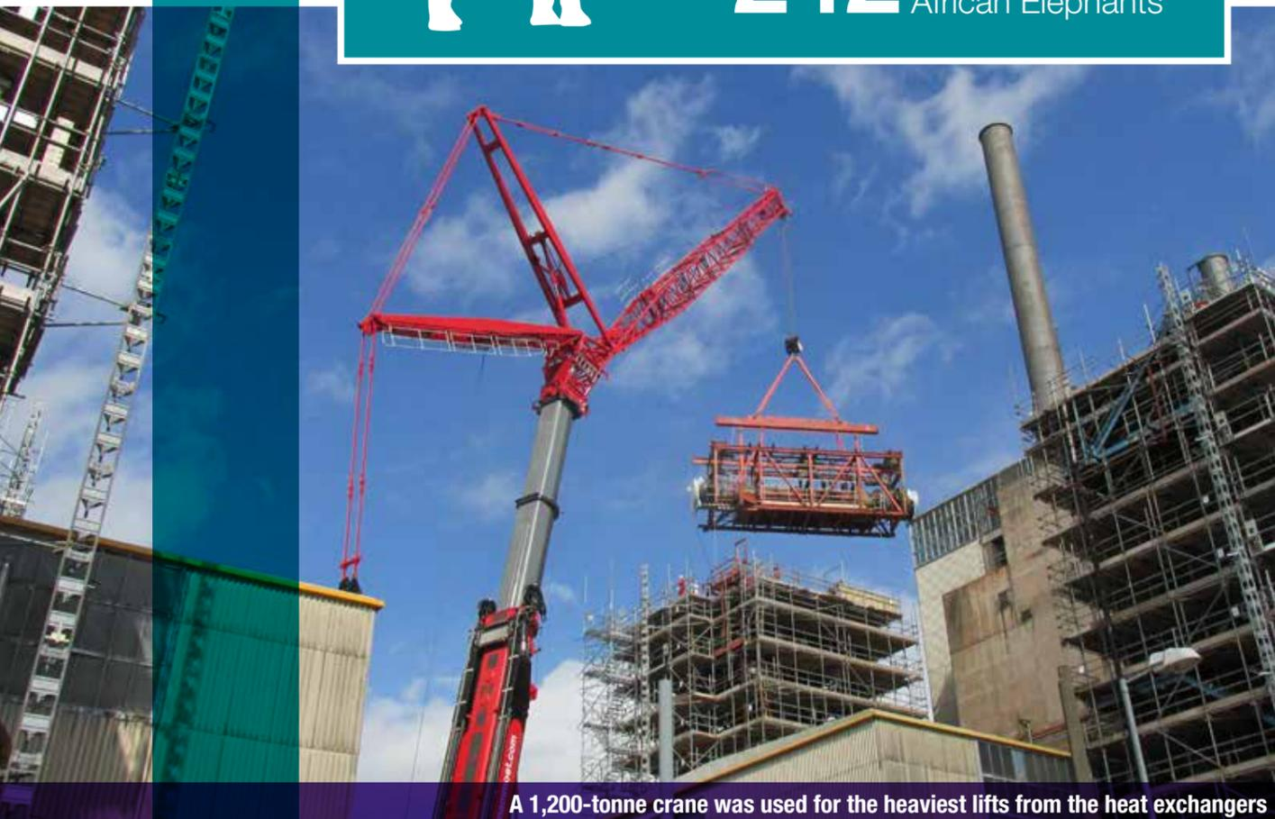
A 1,200-tonne crane was used for the heaviest lifts from the heat exchangers
