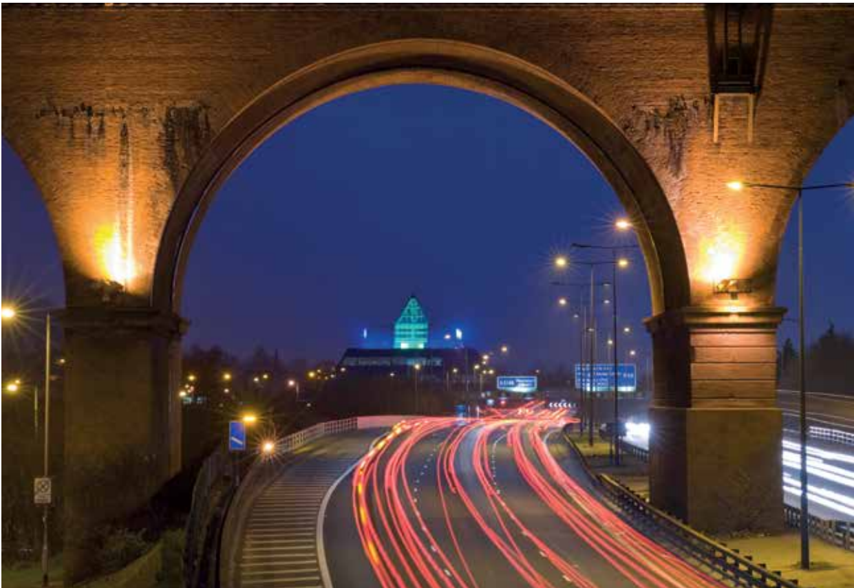
Grade II* listed Stockport viaduct on the M60, North West
