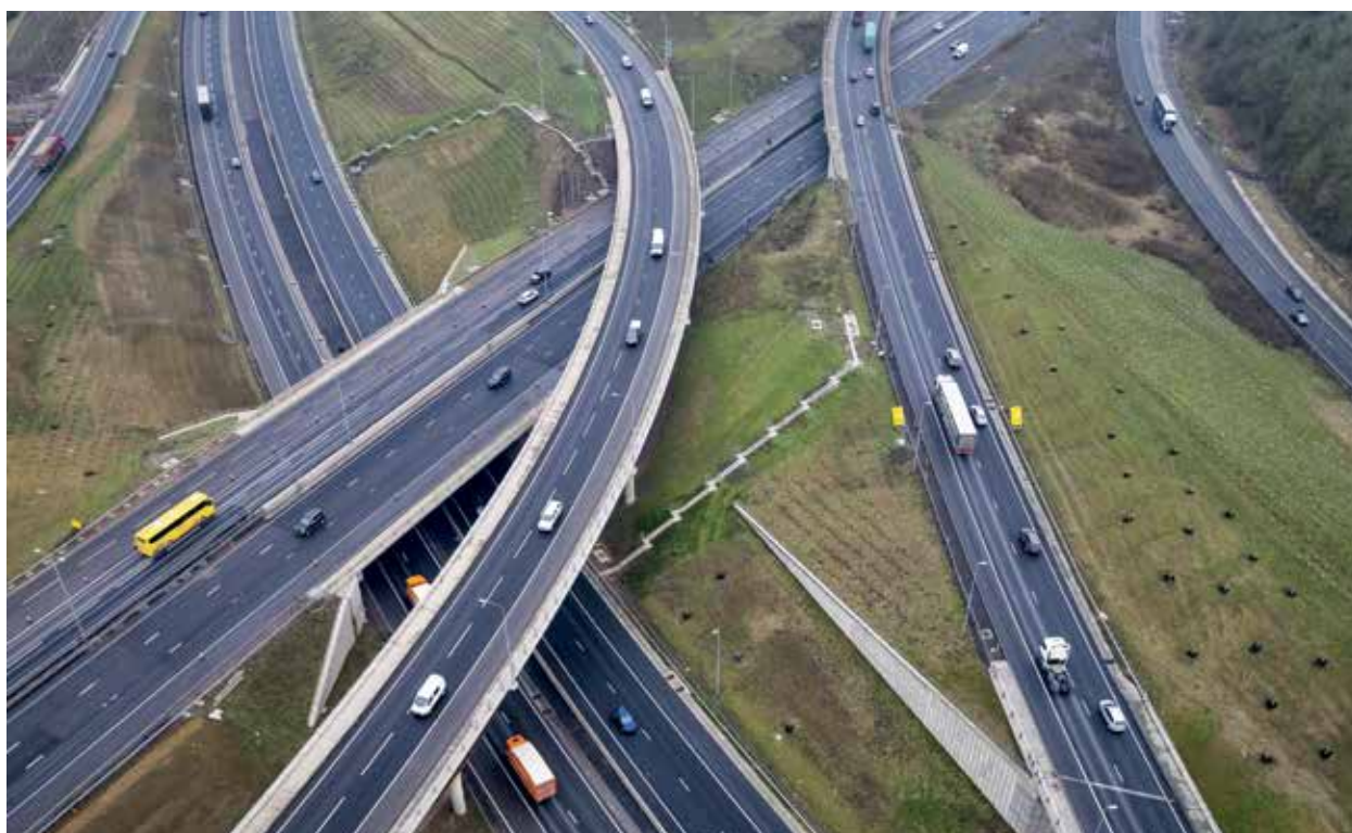
Catthorpe Interchange, East Midlands
