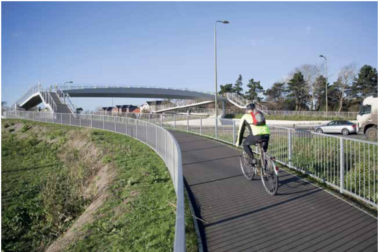
Cycling and pedestrian bridge on the A27
