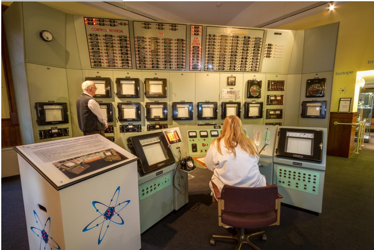
DMTR control room in Caithness Horizons
