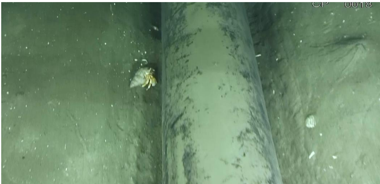
Figure 5-2 – Curlew D Pipeline Exposure Example
