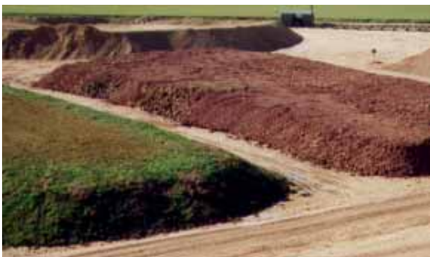
Clearly defined stockpiling of different soil materials
