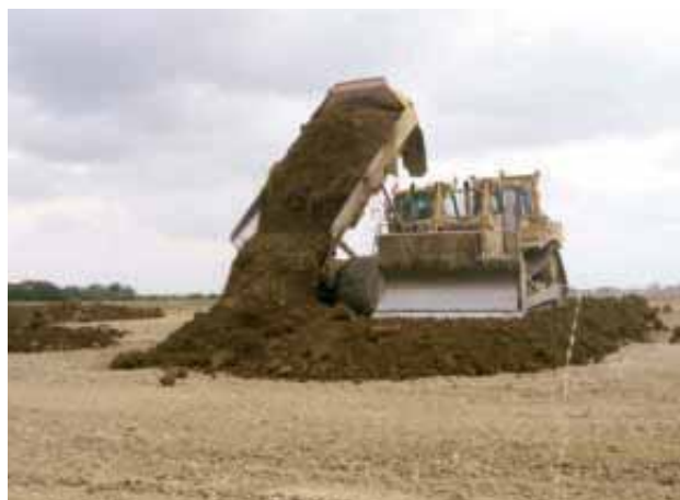
Starting a 'peninsula' of topsoil
