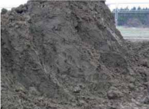
Topsoil stockpiled when wet and plastic
