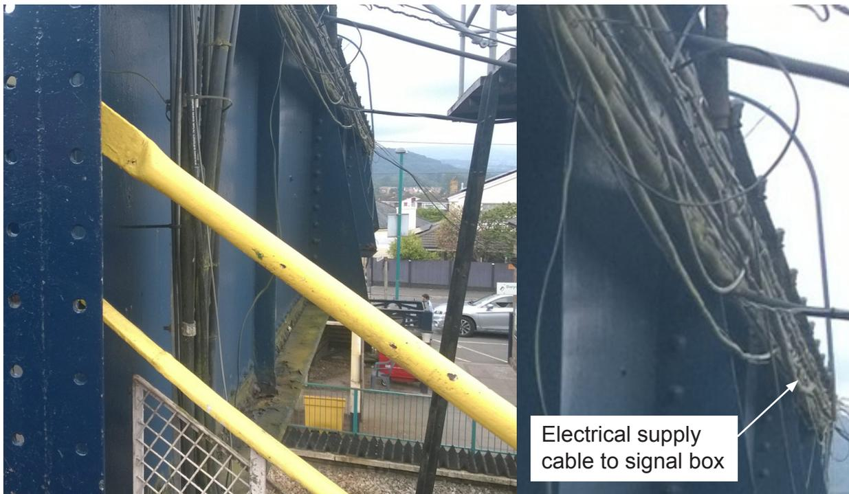
Figure 22: Photograph of the cables and cable tray running over the footbridge at Abergavenny station on 19 July 2017 (images courtesy of Centregreat Engineering)
