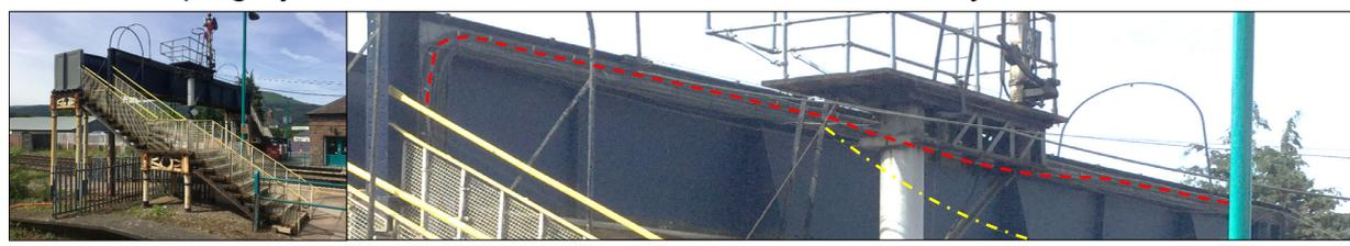
*Figure 7: Images of the electrical supply (highlighted in red) and telecommunications (highlighted in yellow) cables drooping from the footbridge from February 2016 to July 2017 (images courtesy of Network Rail)*
