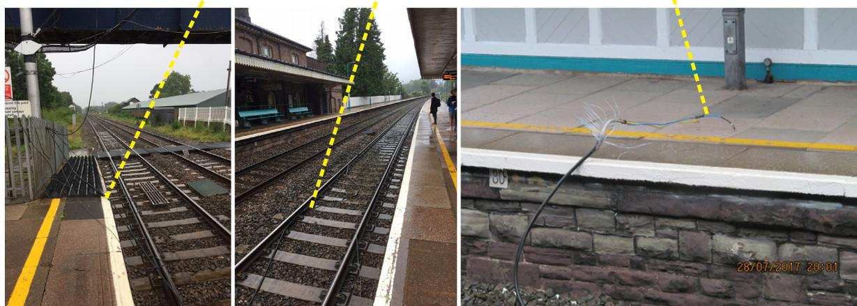
Figure 12: Diagram and photographs showing the position of the electrical supply cable after it came to rest (left and middle images courtesy of Network Rail, right image courtesy of British Transport Police)
