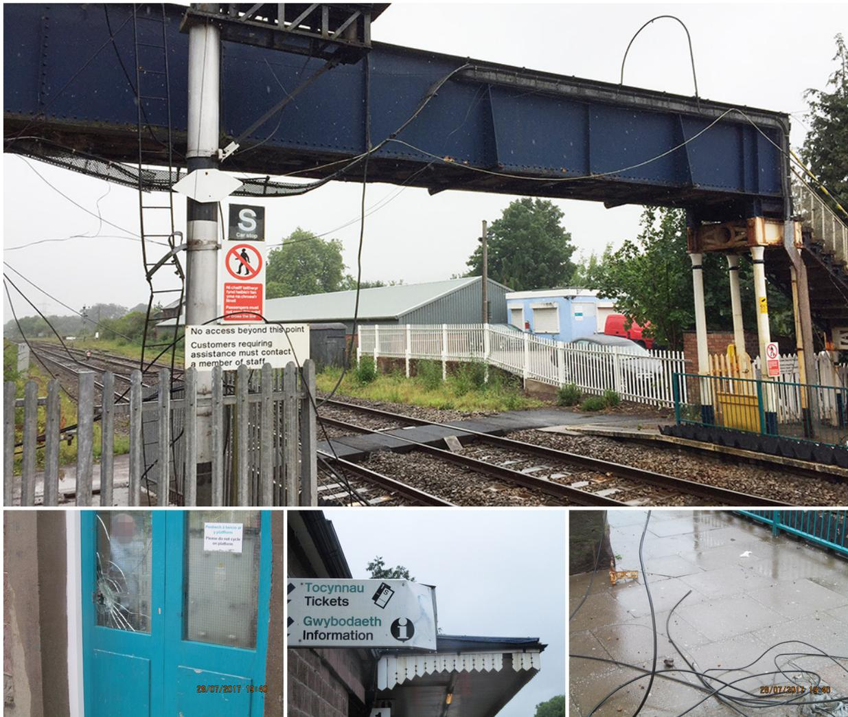
Figure 2: Damage to the cable tray running over the footbridge, station buildings and to other equipment on the station (main image courtesy of Network Rail and inset images courtesy of British Transport Police)
