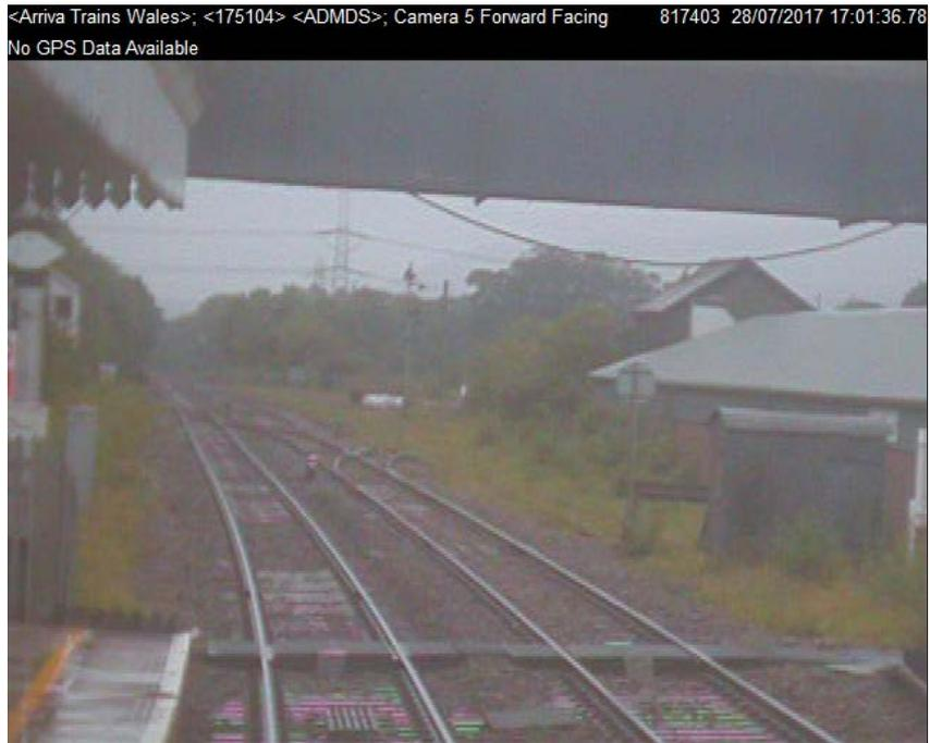
Figure 1: FFCCTV footage from a preceding train, showing the drooping power cable.
