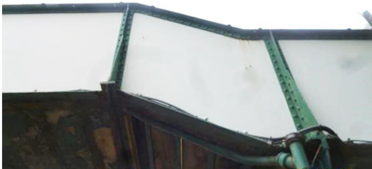
*Figure 24: Cables routed on the outside of the footbridge at Helsby station (image courtesy of Network Rail)*
