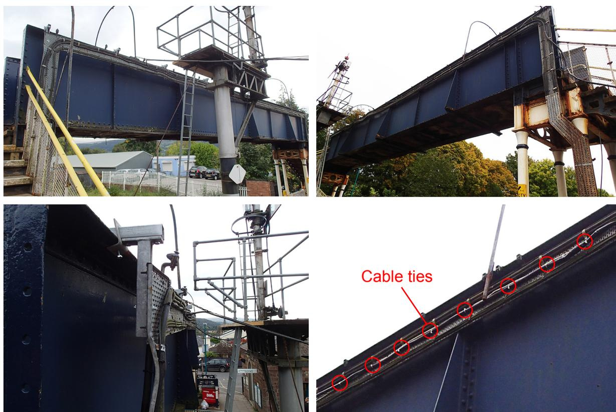
Figure 23: The repairs made to the footbridge cable tray after the accident
