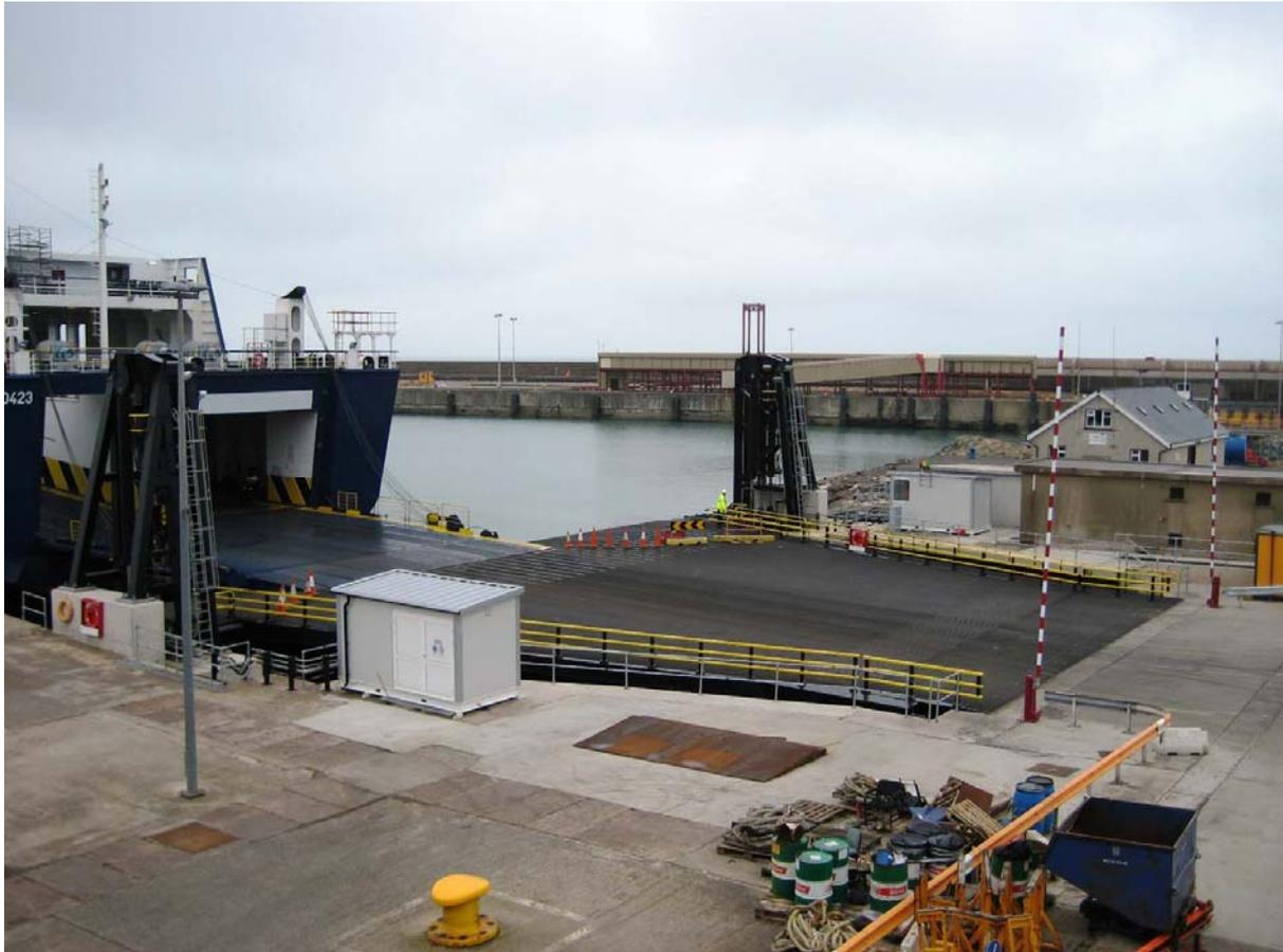
**Figure 2.11 Typical linkspan**
